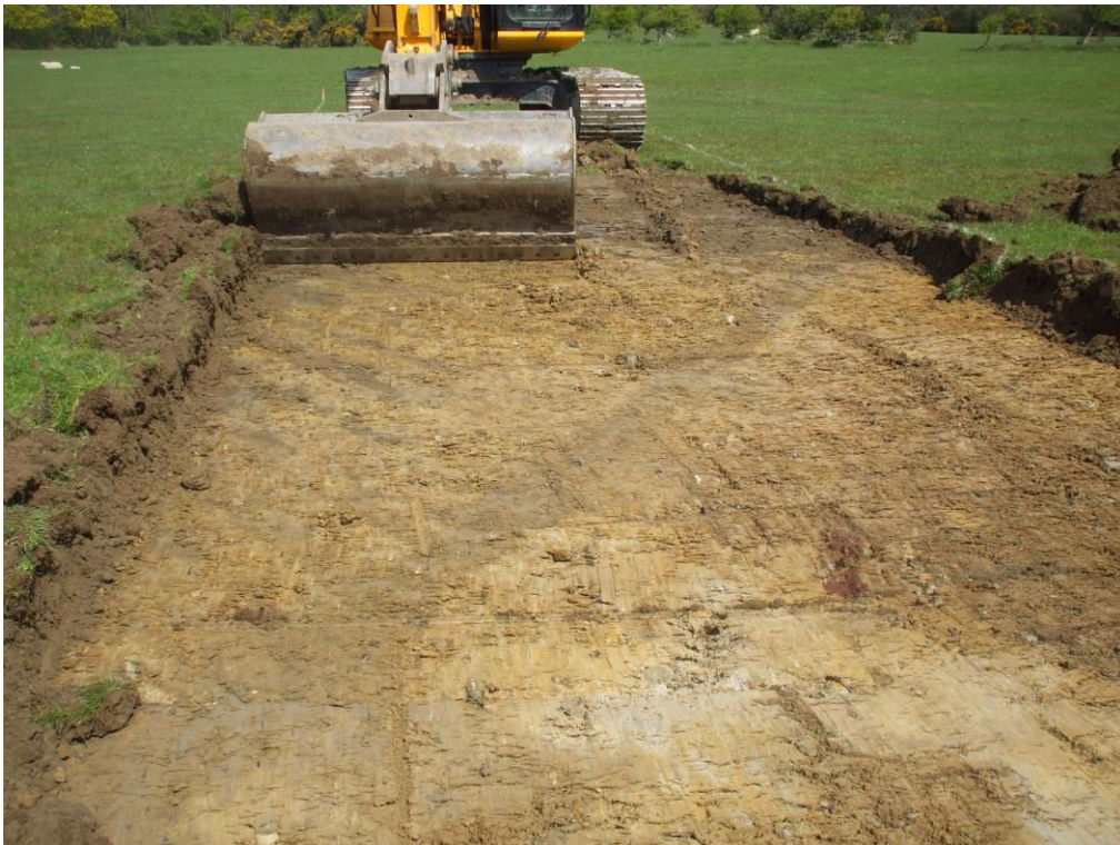
Plate 2 - Working shot of haul road showing field drain
