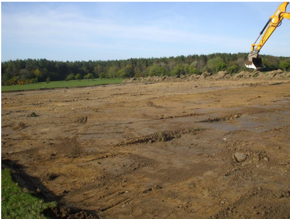
Plate 1 - Turbine 1 crane pad stripped
