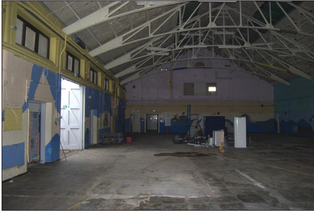
PLATE 3: Drill Hall, Looking Southwest
