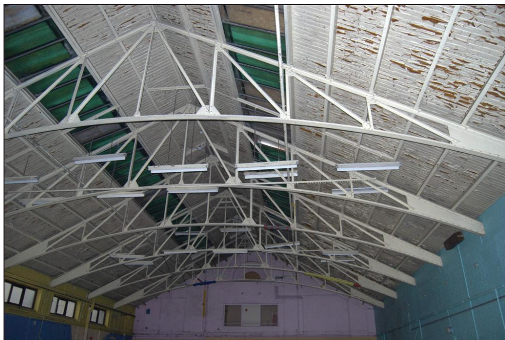
PLATE 4: Drill Hall Roof
