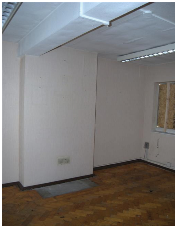
PLATE 10: Room F8, Chimneybreast and Floor
