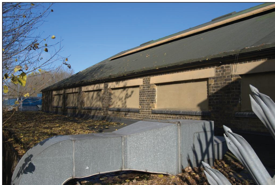
PLATE 2: External View, Looking North
