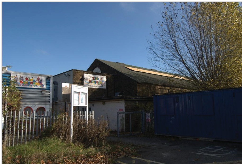
PLATE 1: External View, Looking East
