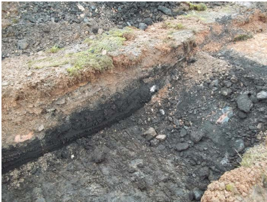
Plate 4 - West-facing section of Trench 19 showing made ground over peat
