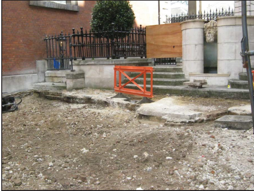
Plate A. Features [11], [12] & [13] Looking North
