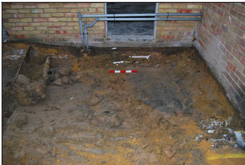
Plate B. Trench 2 Looking West
