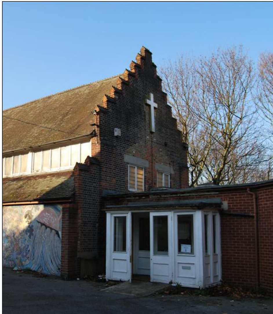
Plate 3: East End Of Hall, Showing Repairs
