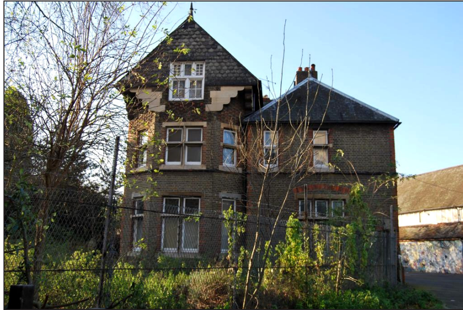
Plate 13: The Vicarage, Looking West
