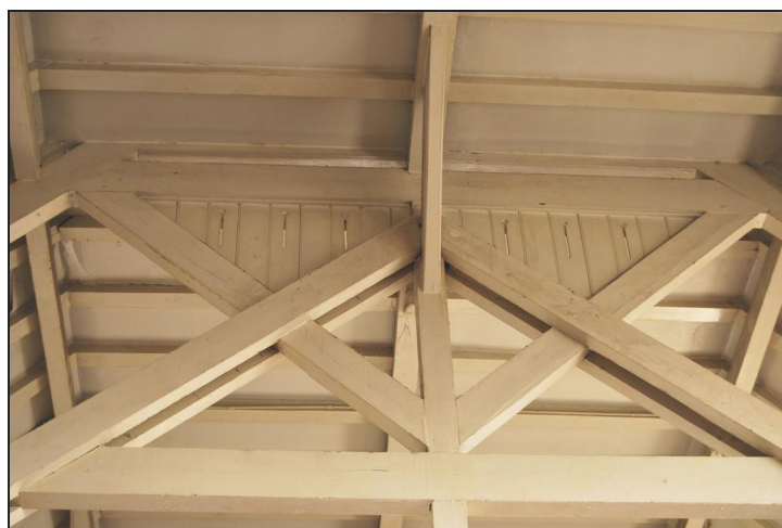
Plate 5: Boards At Truss 'E'.
