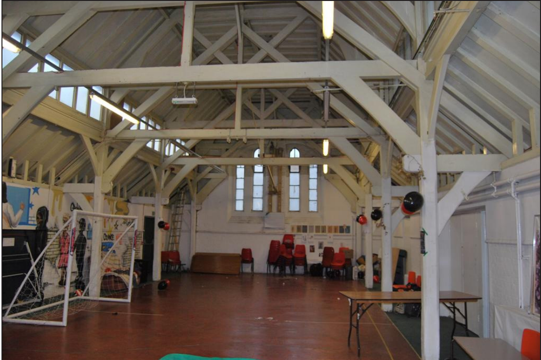
Plate 4: View Of The Hall, Looking West
