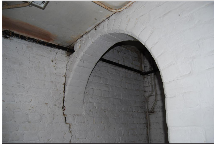
Plate 11: Structural Crack
