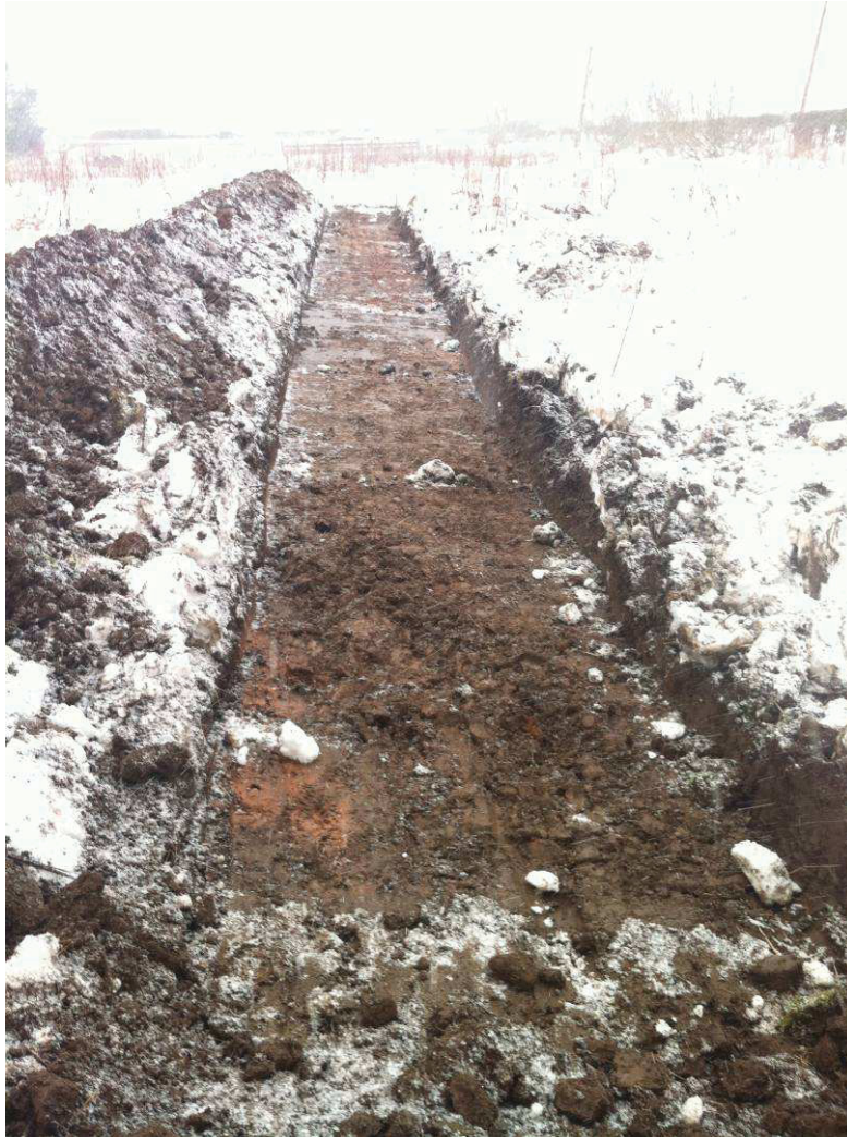
Figure 2 View of Trench 1
