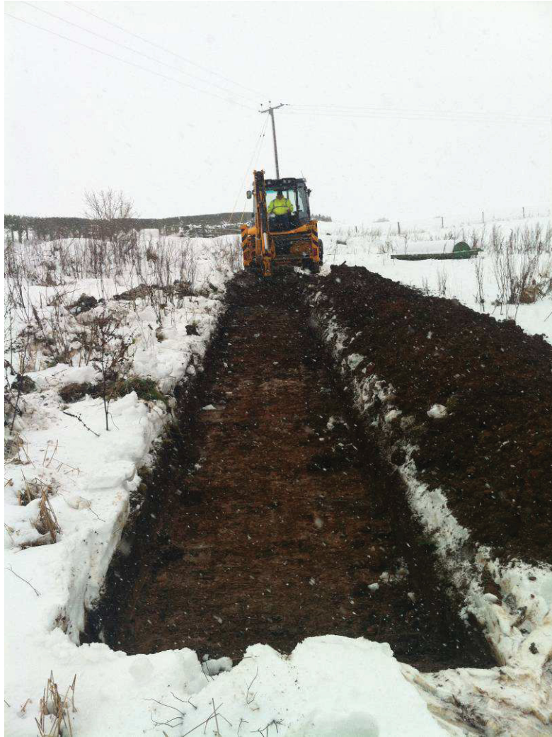
Figure 1 View of Trench 1 Under Excavation
