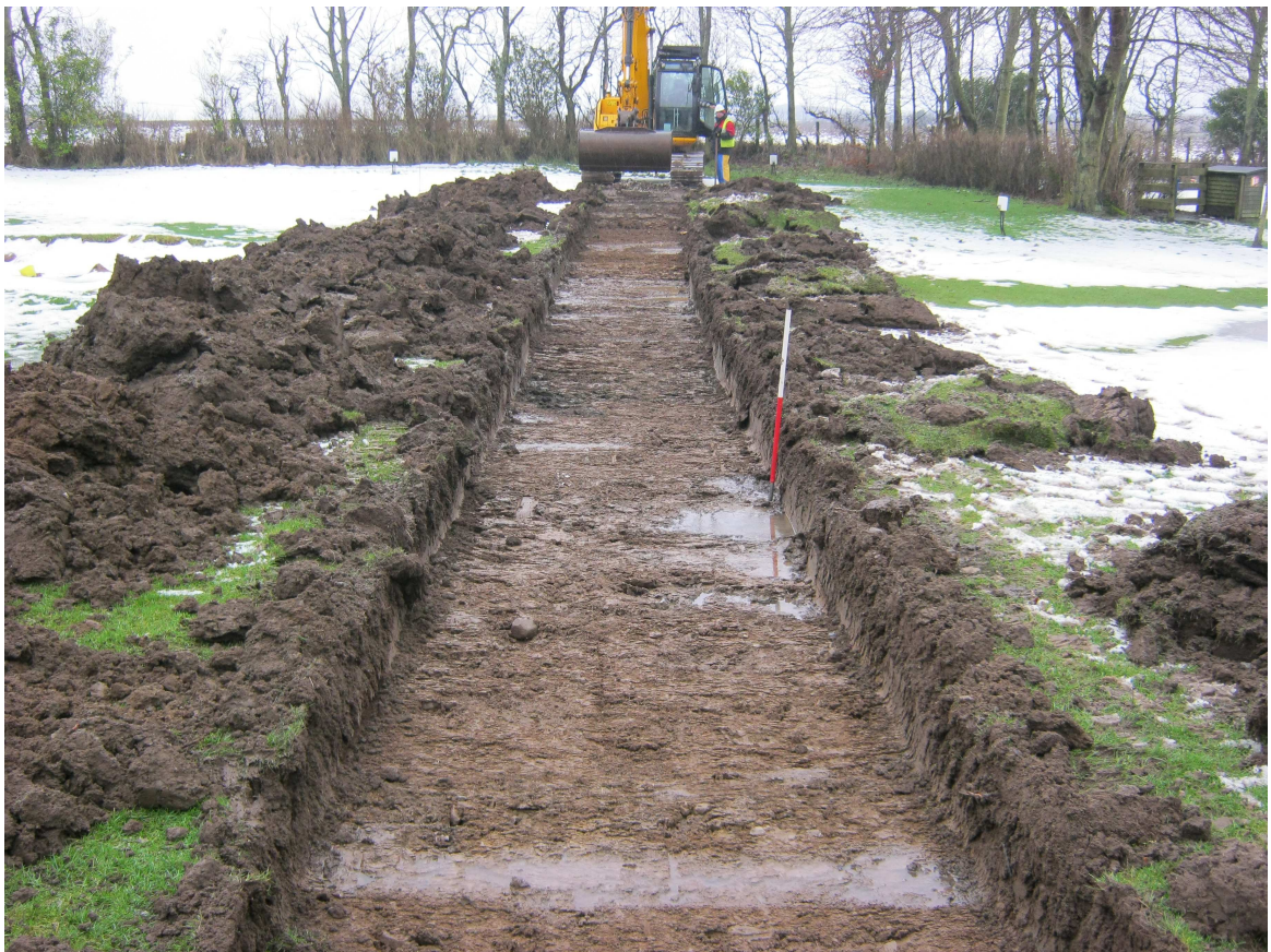
Plate 1 Trench 1 post-excavation from north-east
