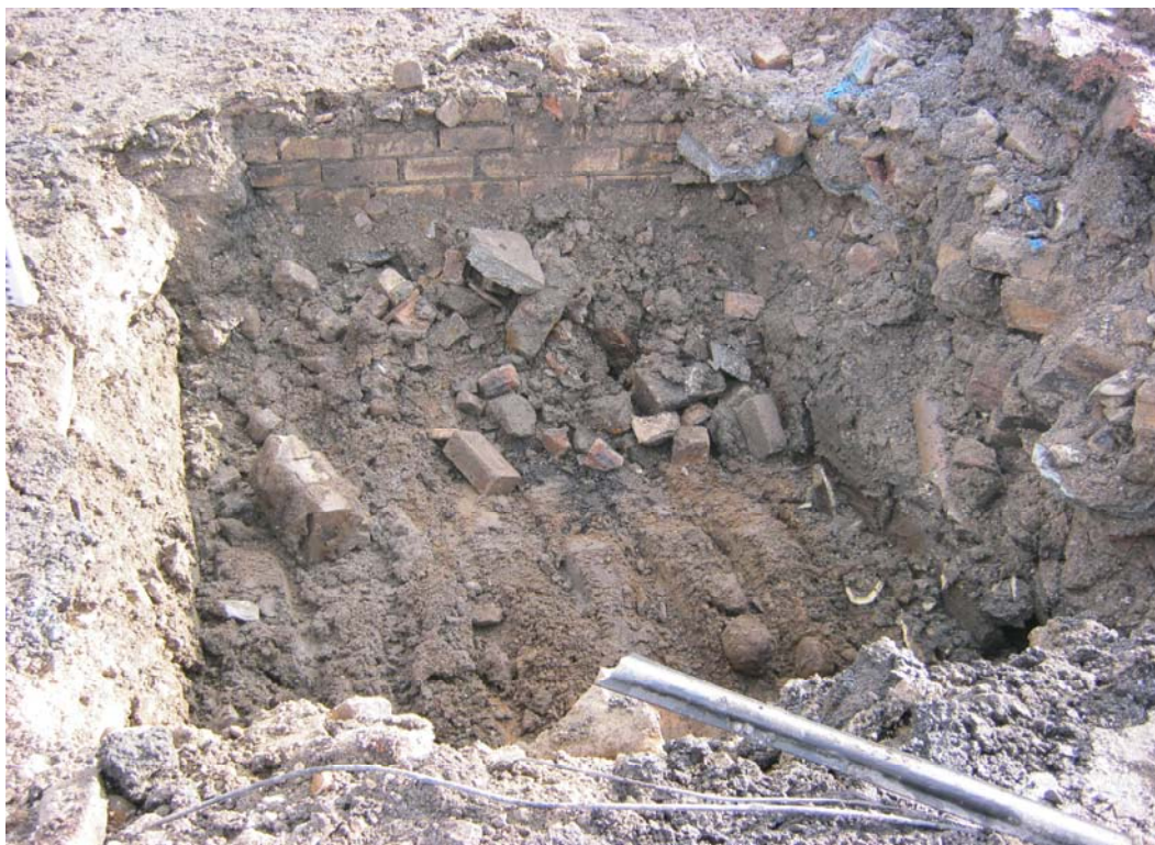
Plate 4; Foundation pit along frontage from south
