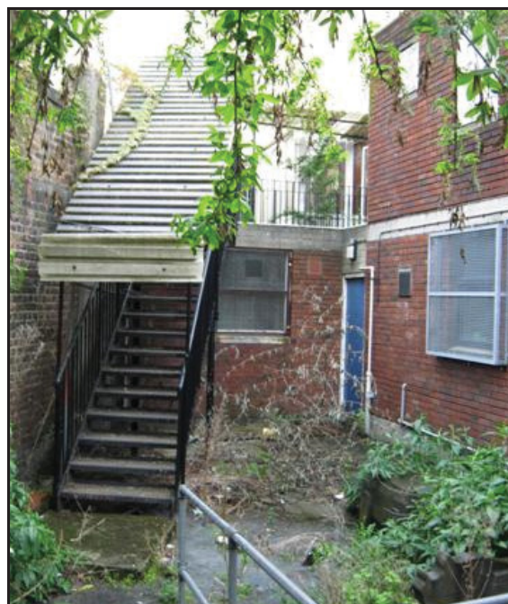
PLATE C: View of yard area from the west
