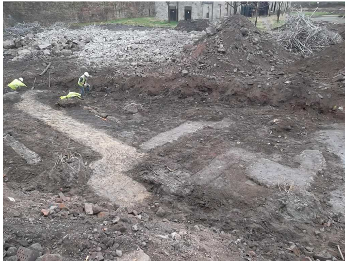
Plate 2 - SW end of Structure 1 foundations
