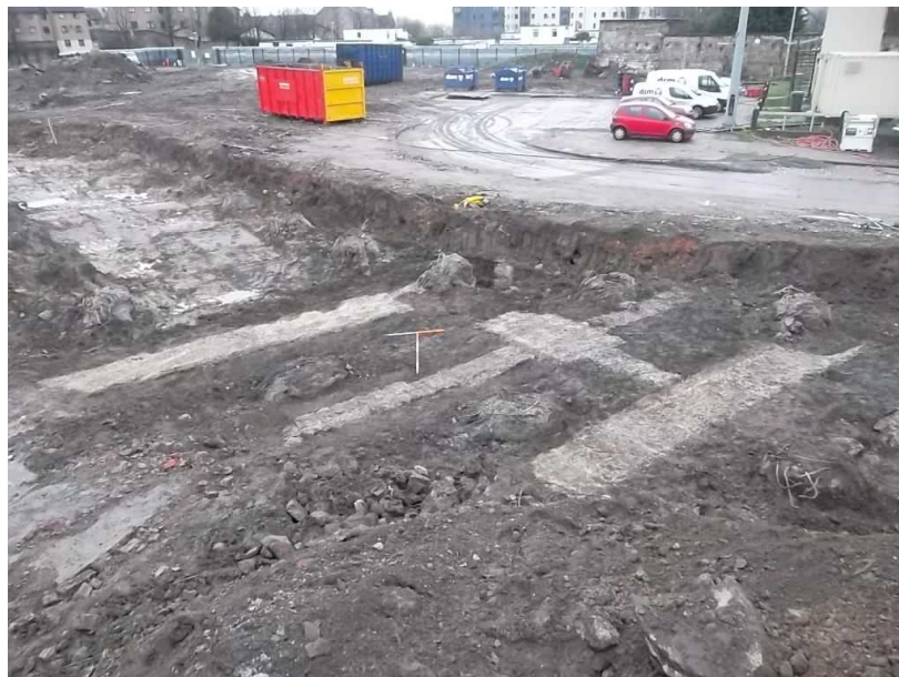
Plate 1 - NE end of Structure 1 with wall [007] through centre
