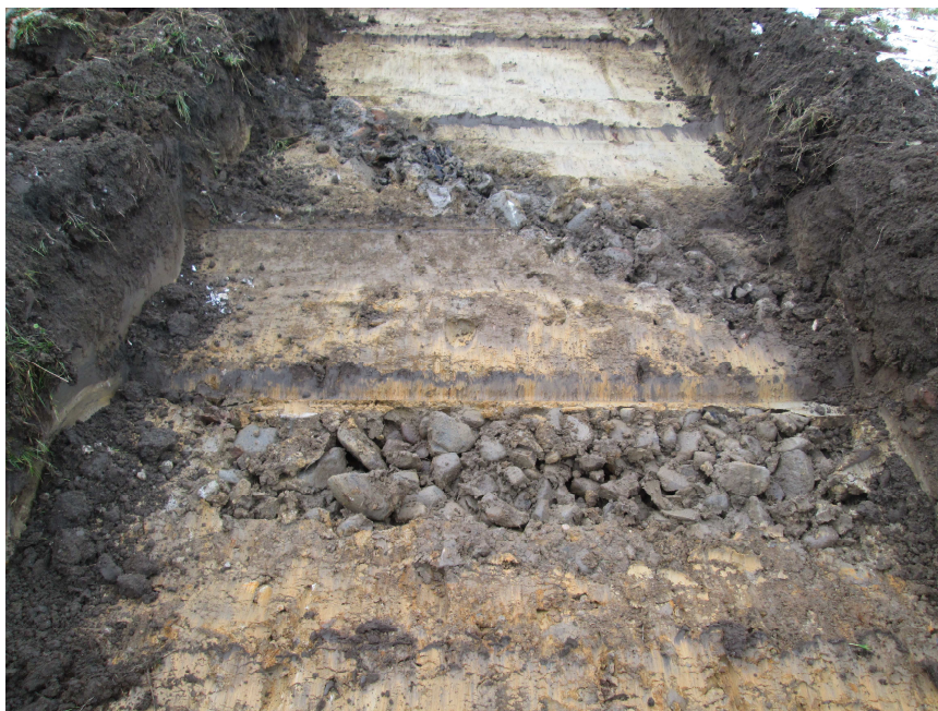
Plate 2 - Trench 31 showing two stone filled drains
