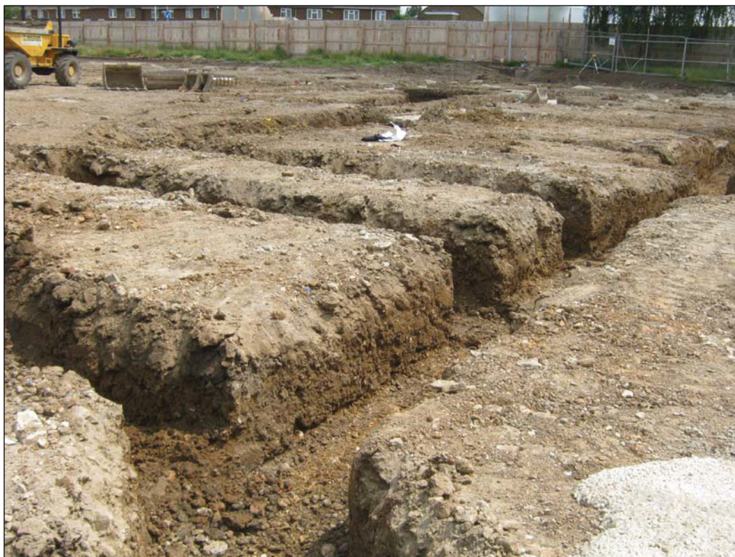
Plate B: Foundation trenches in NW area of the site.
