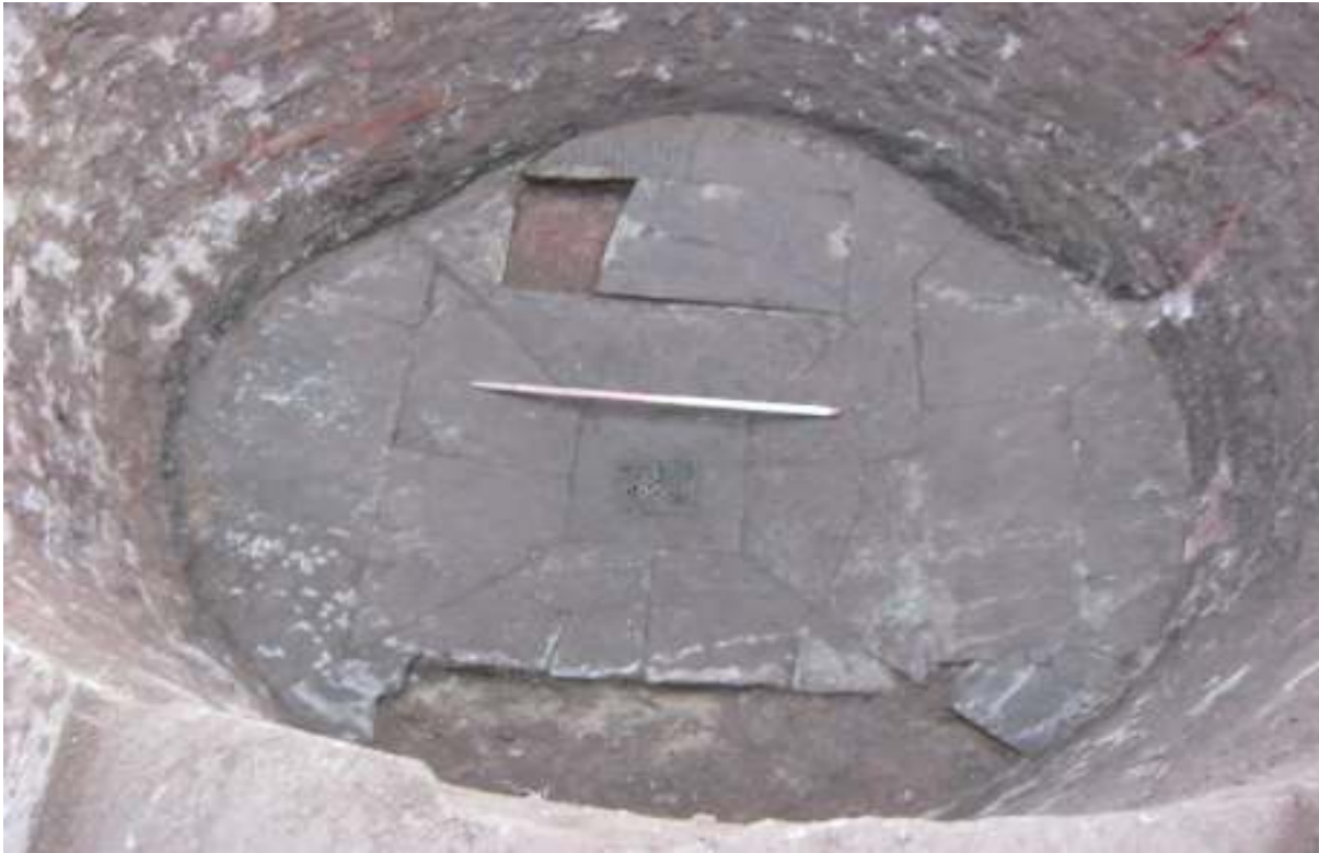
Plate 7 – The floor of the Ice House chamber showing central grate
