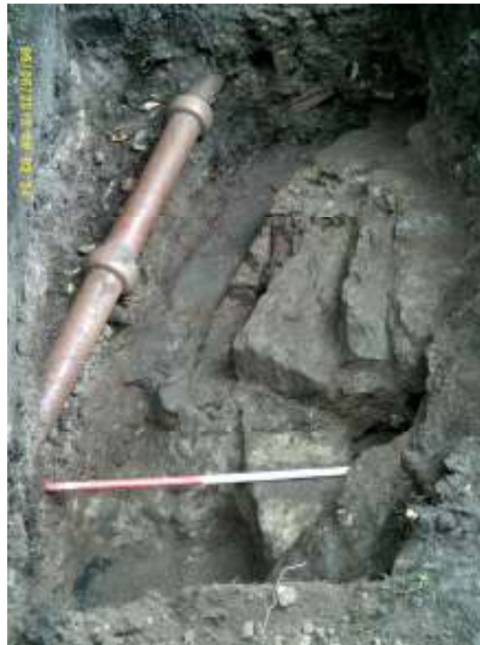
Plate 3 - Corbelled roof and supporting wall of Ice House
