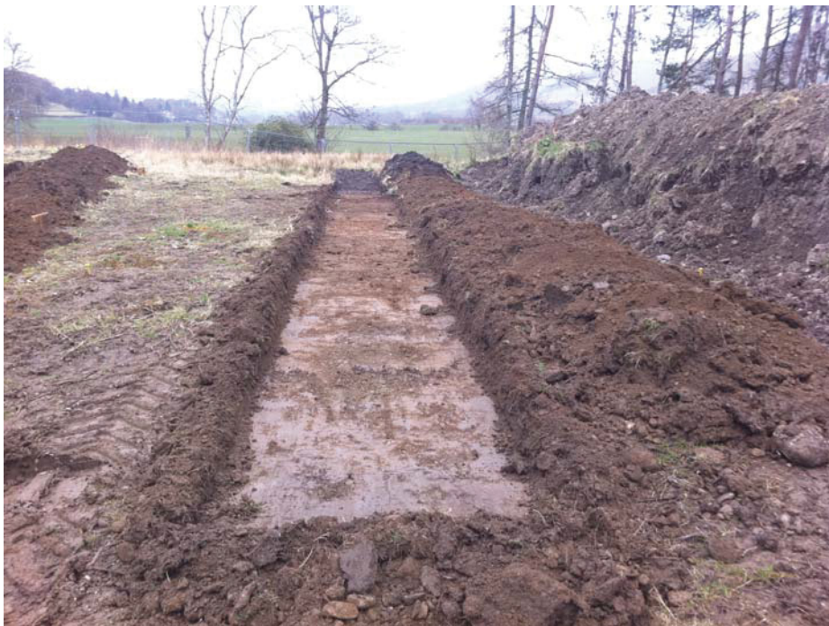
Plate 1 - Trench 1 Post-excitation showing topsoil bund to east
