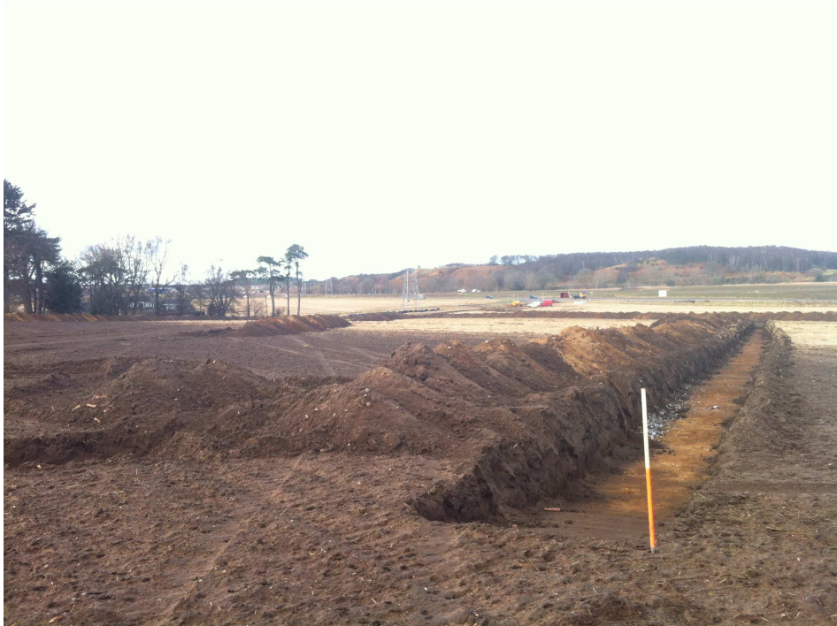
Plate 1: General view of open trenches
