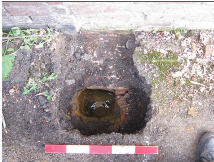
Plate 2: Ground Investigations Test Pit 9 looking south
