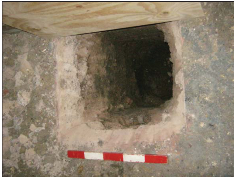
Plate 3: Ground Investigations Test Pit C looking east
