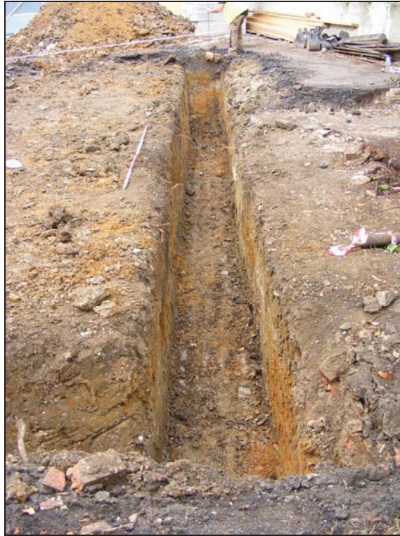
Plate 6: Northern side of foundation trench looking west
