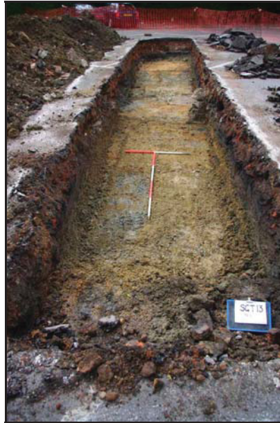
Plate A. Trench 1 Looking Northwest
