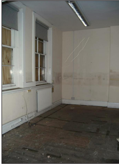
Plate 18: Room 2 Looking Northwest
