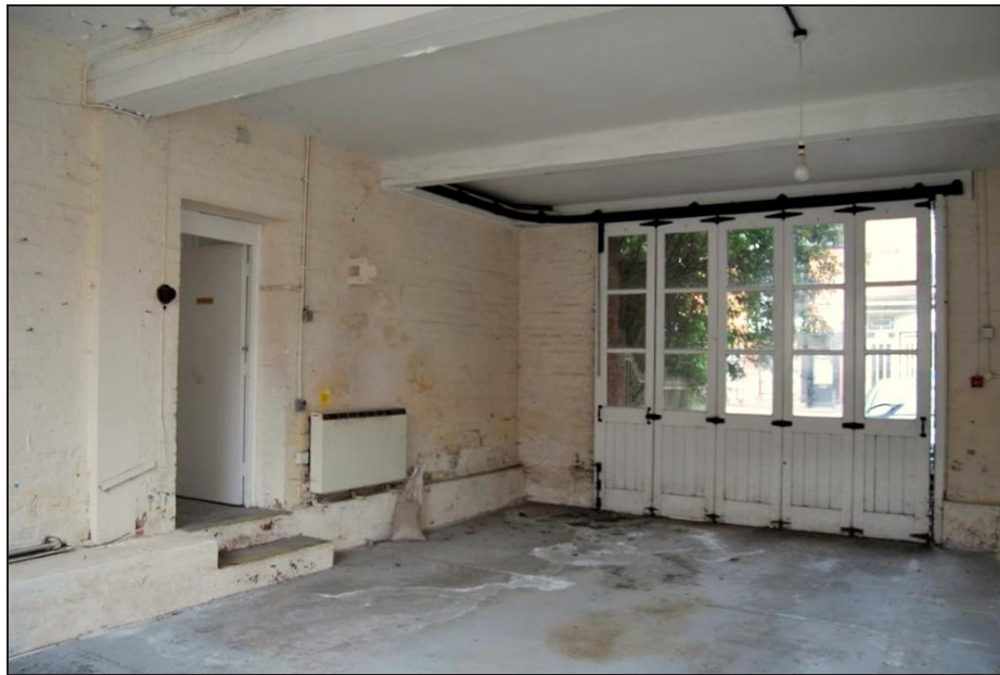
Plate 8: Room 1 Looking West
