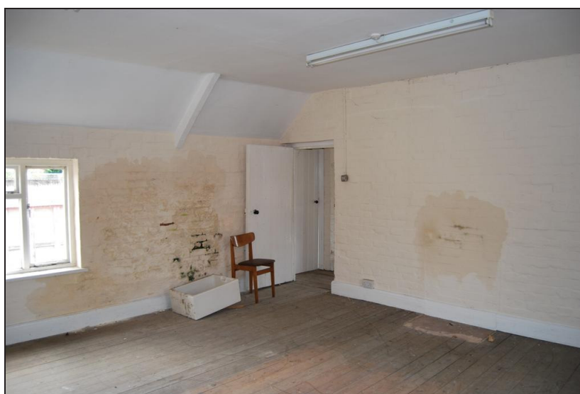
Plate 10: Room 6 Looking Southwest
