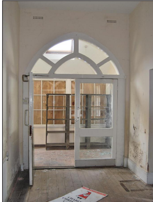
Plate 15: Doorway between Porch (Room 1) and Hall (Room 17)
