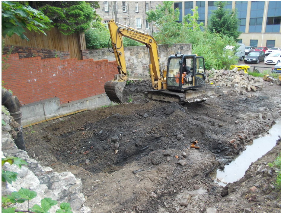
Figure 1 Excavation of Foundation Trenches
