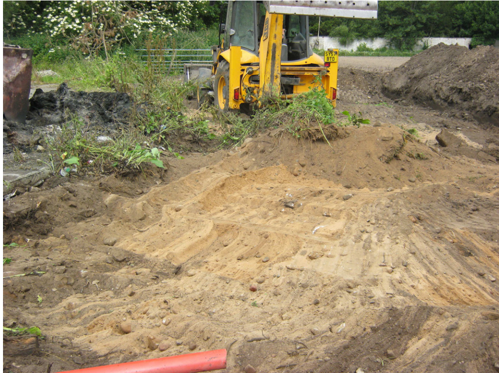
Plate 2. Site during Monitored Topsoil Stripping from west
