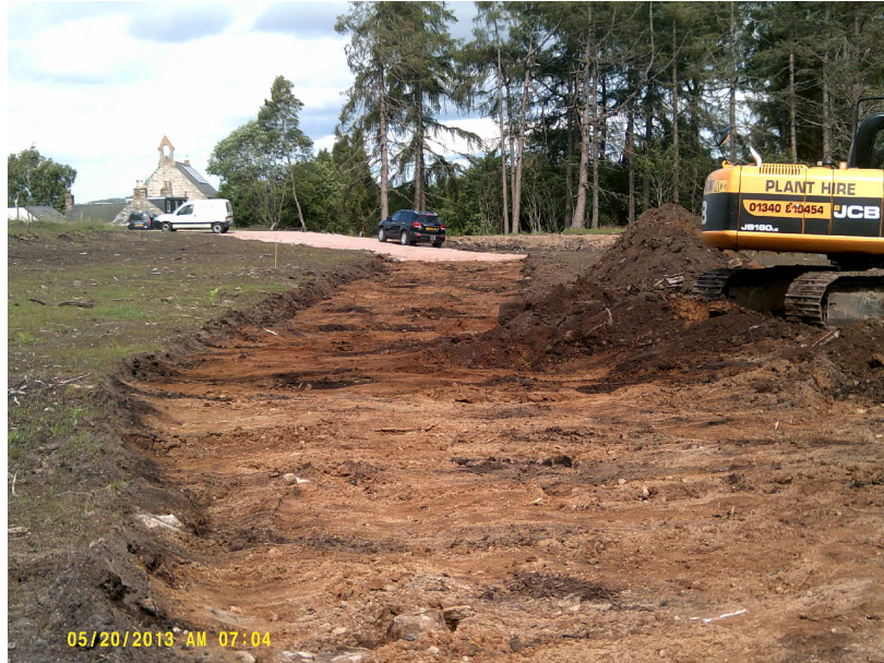
Plate 1 - Driveway stripped showing root bowls from forestry
