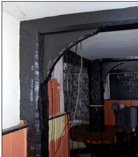
Plate 6: Detail of Post and Beam Assembly. Carpenter's Mark at Joint.
