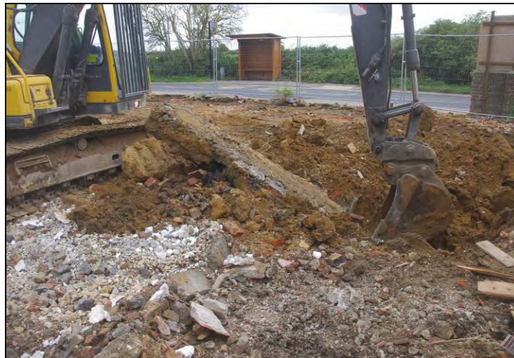
Plate 1: Removal of the footings
