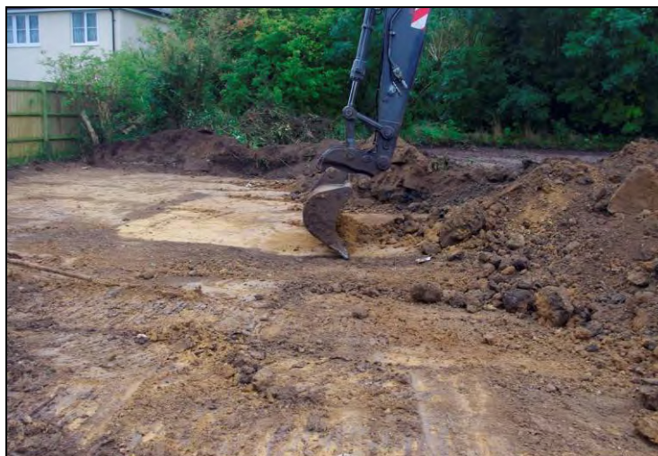
Plate 2: Reducing the ground
