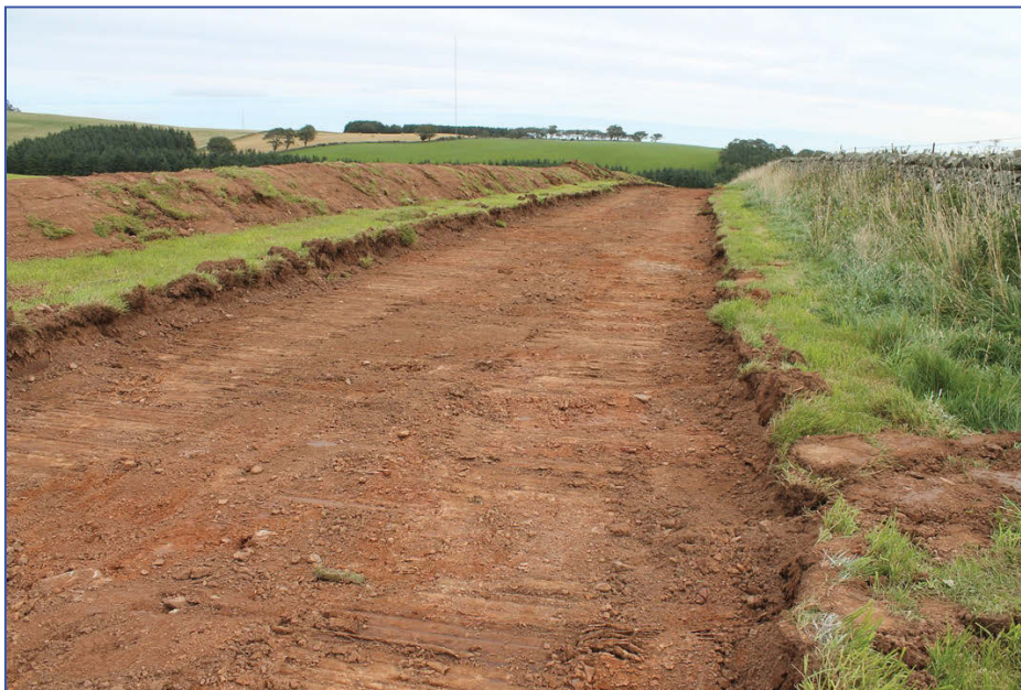
Plate 1: General view of the stripped access road from the north
