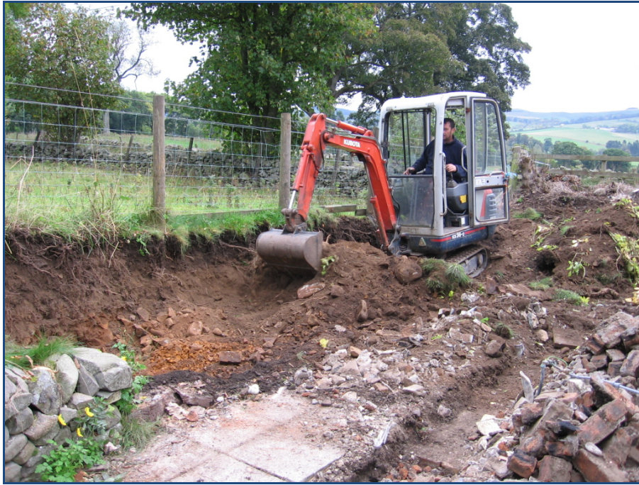
Plate 1: Removal of bank on northern edge of development area showing terracing of garden.
