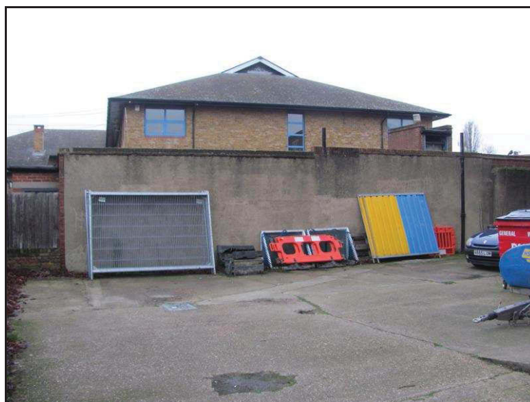
PLATE J: Northern part of site showing boundary walls with Grade II Listed Elmfield / Tiffin School (AOC 96) (direction north)
