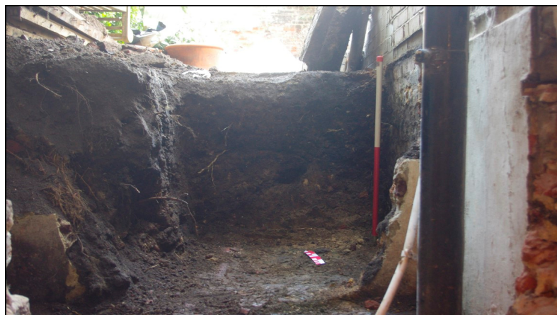
Plate 2: Section of foundation trench looking southeast
