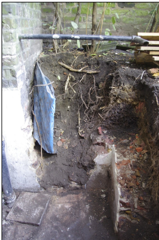
Plate 1: Area excavated for steps to basement looking southwest
