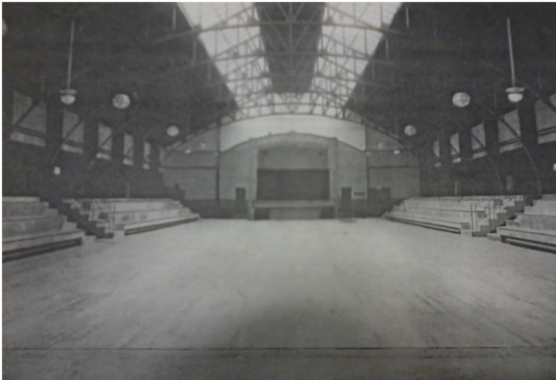
With the floor in place
