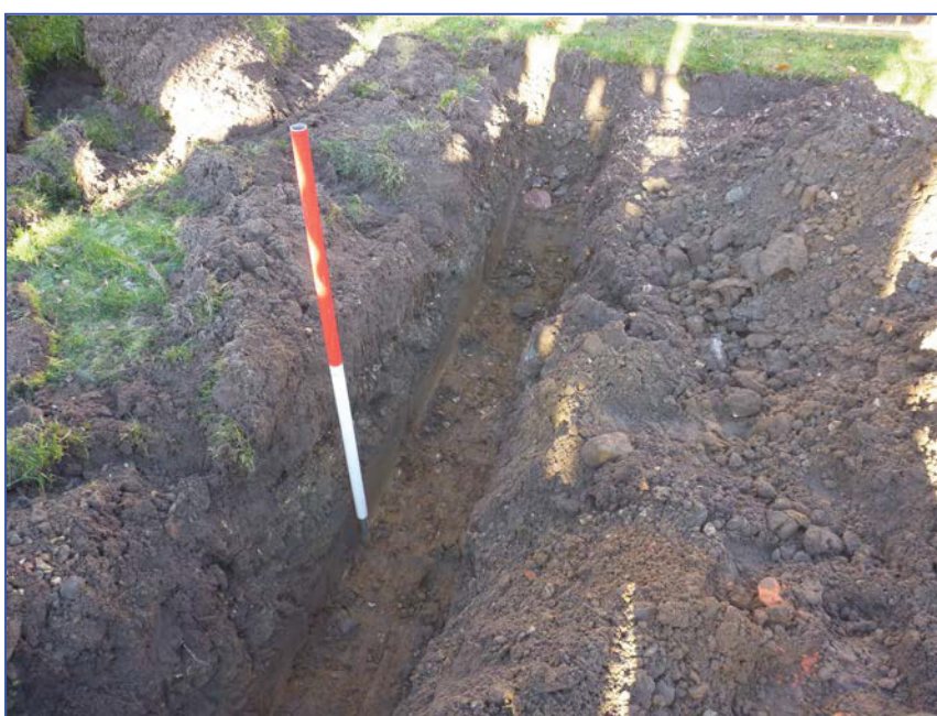
Plate 1: General view of the eastern foundation trench
