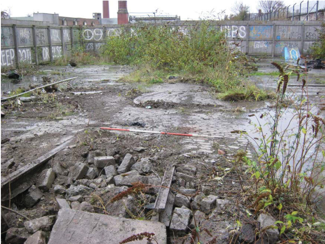
Plate 2: View of relict cobbled road [002] and rails [001]
