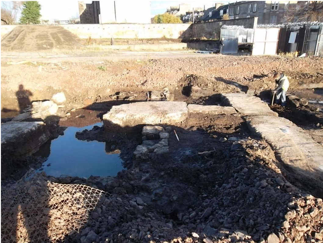
Plate 19 - Concrete foundations in Area E2
