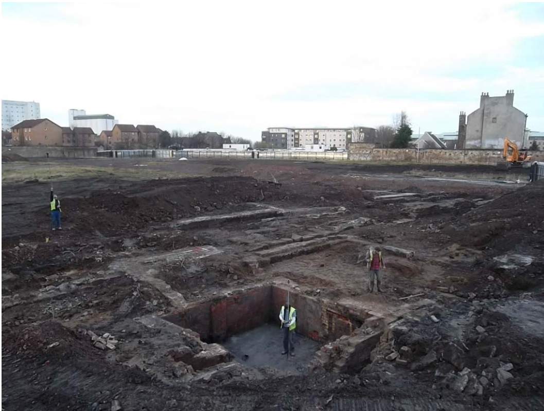
Plate 21 - General shot showing boiler room and surrounding foundations
