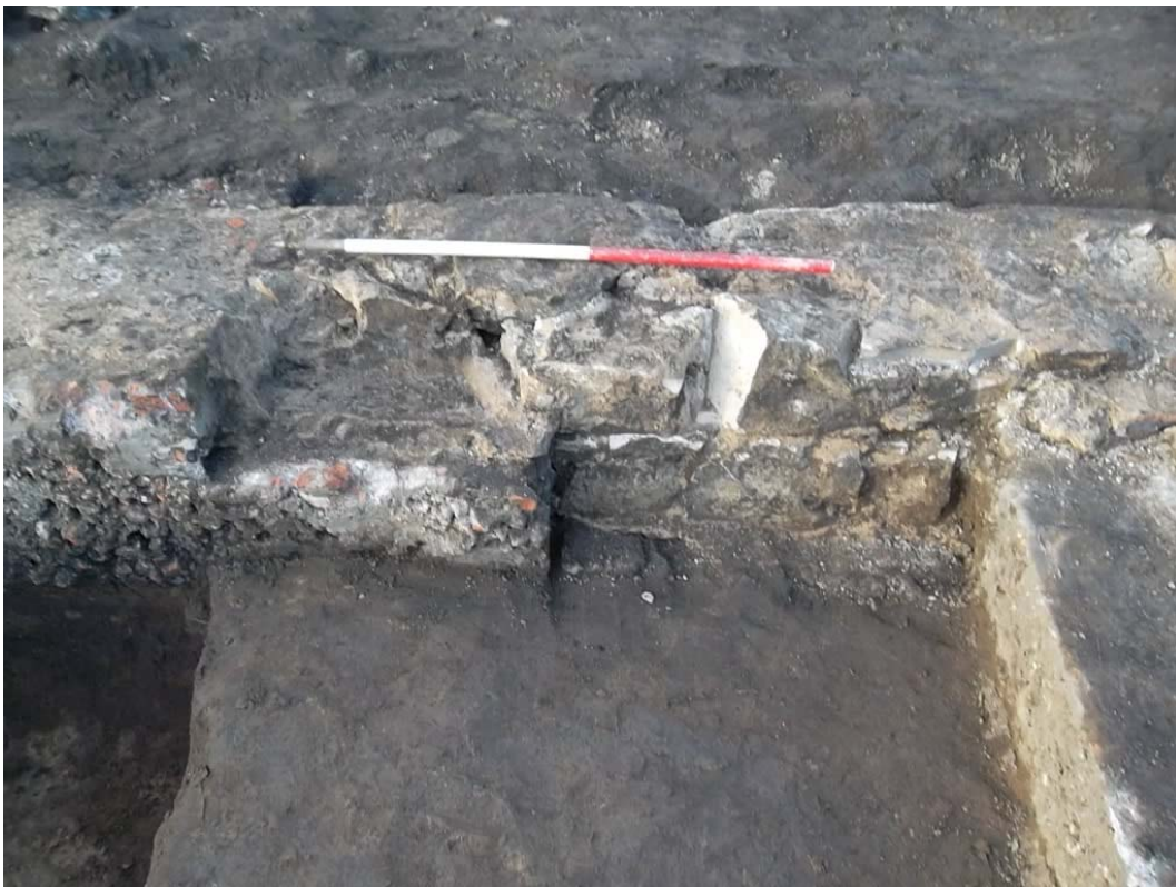
Plate 6 - View of concrete foundations [100] abutting sandstone wall [101]
