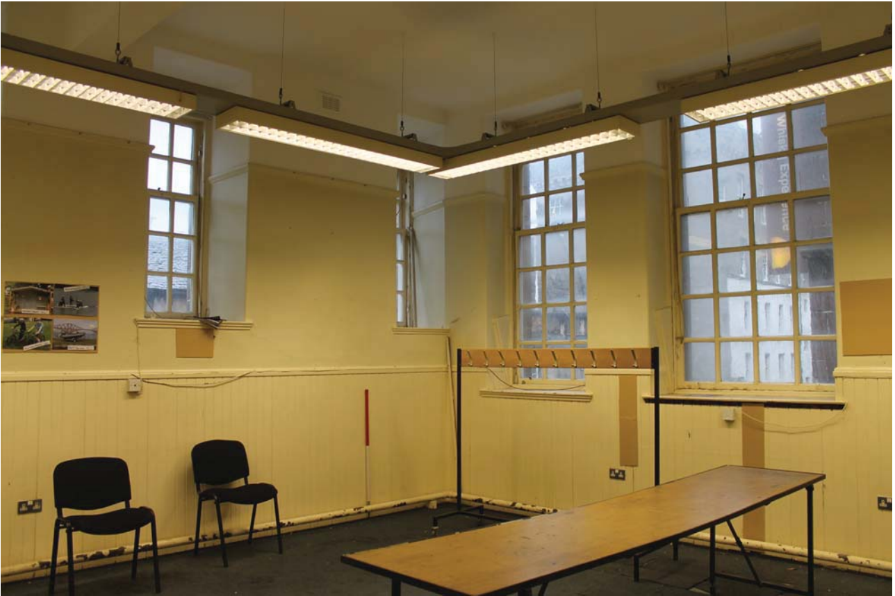
Plate 5: Cannonball House, ground floor, general view of the westernmost office from the south-east
