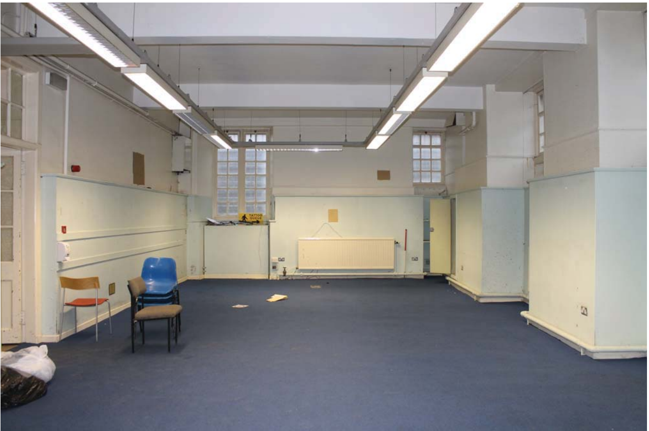
Plate 2: Cannonball House, lower ground floor, general view of the westernmost room from the north
