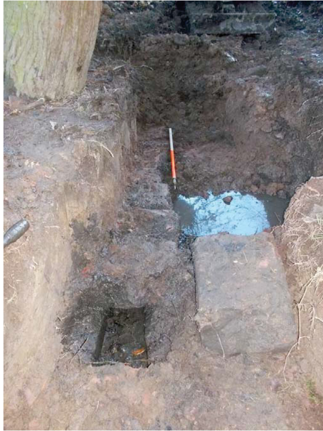
Plate 11: Detail of exposed stone culvert [026] from the west
