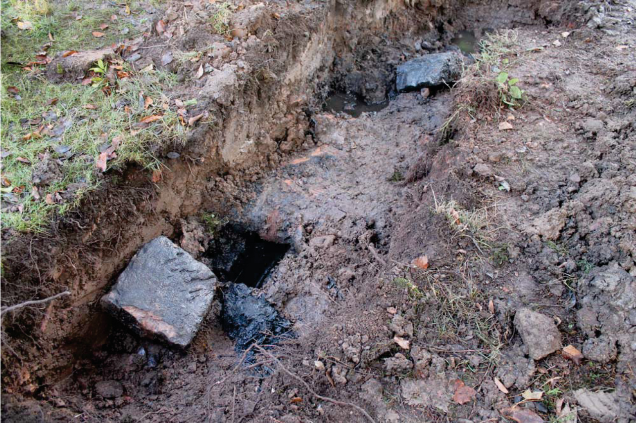
Plate 9: Detail of exposed stone culvert [026] from the west
