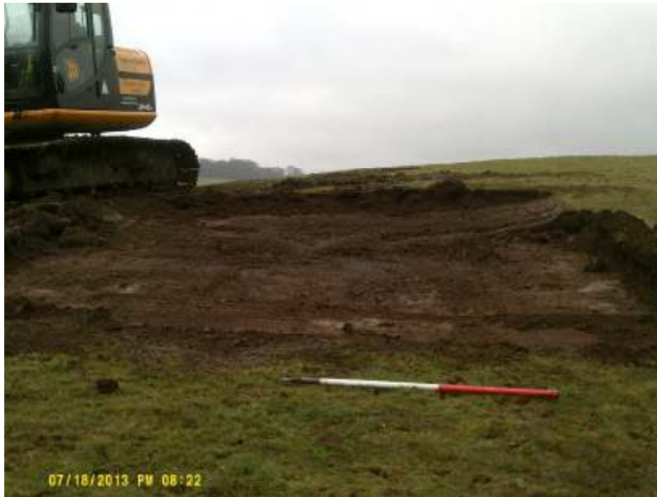
Plate 1 - Post-ex shot of turbine base
