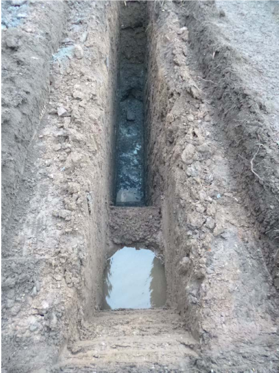
Plate 2: Showing weathered bedrock at base of Trench 1
