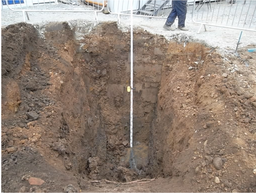
Plate 3: Showing cast iron water main
