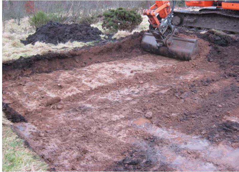
Plate 2 Western end of base under excavation from south-east
