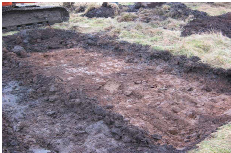
Plate 1 Eastern end of base under excavation from south-west
