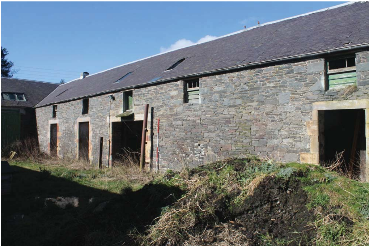
Plate 28: Barn A2, south elevation, general view from the south-east
