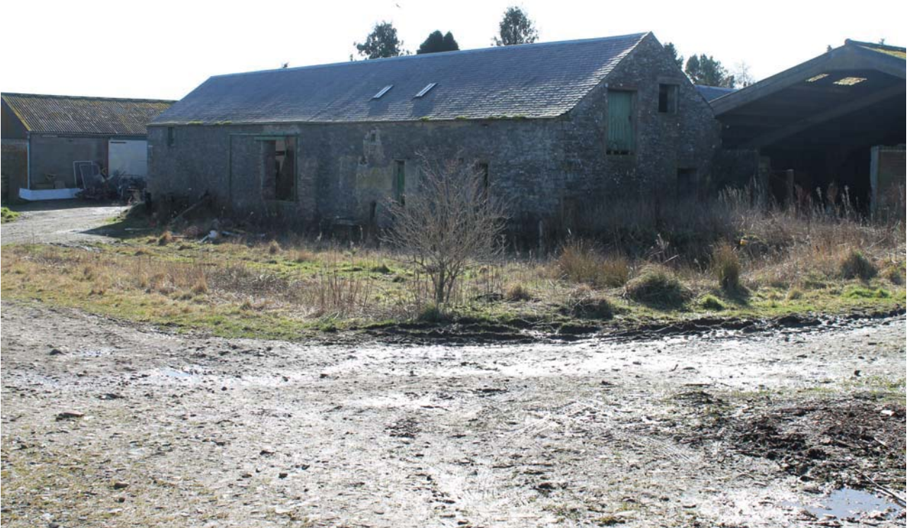
Plate 2: Barn A1, general view from the north-east
