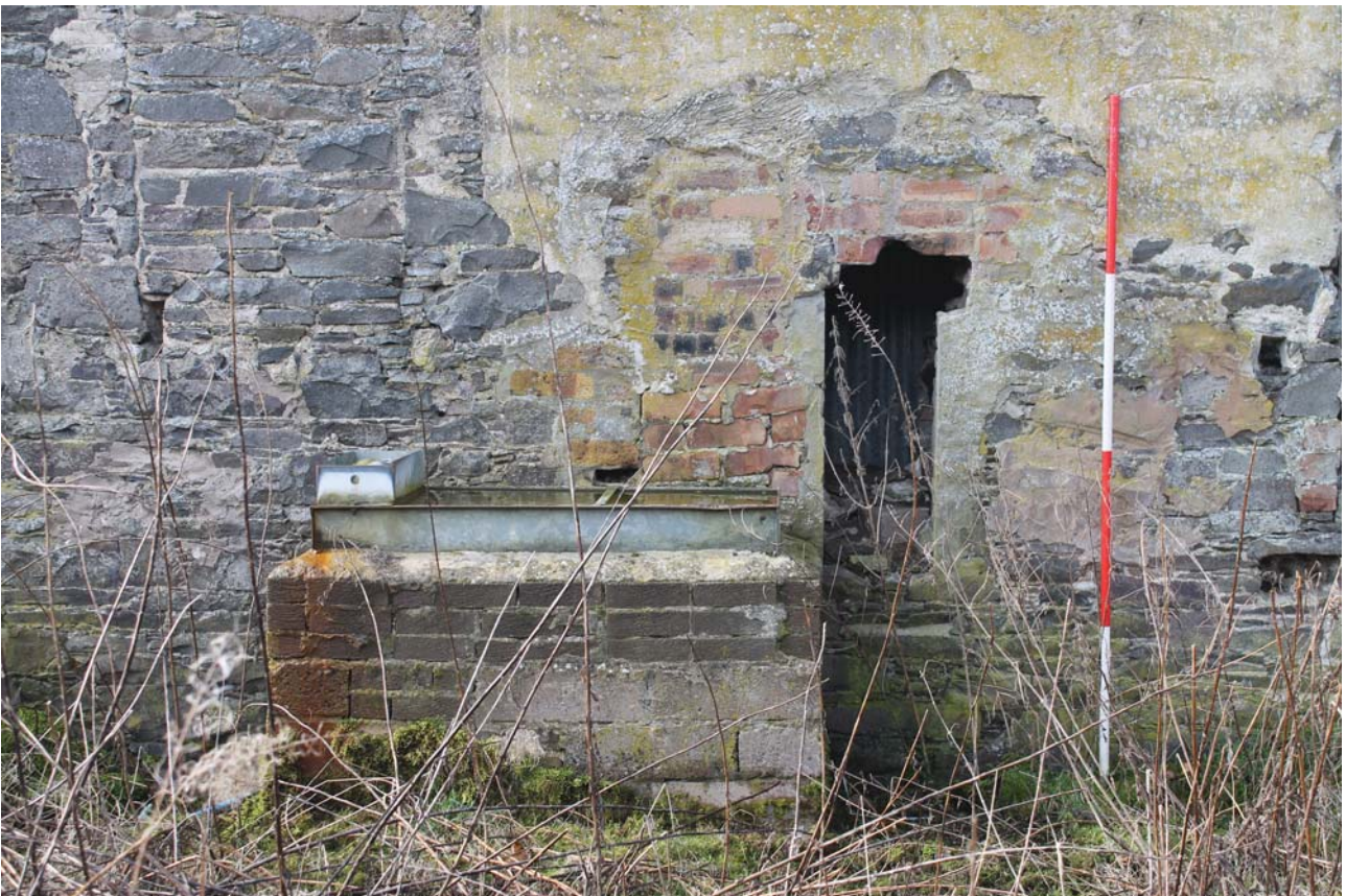
Plate 6: Barn A1, east elevation, detail of the small opening relating to the water wheel from the east
