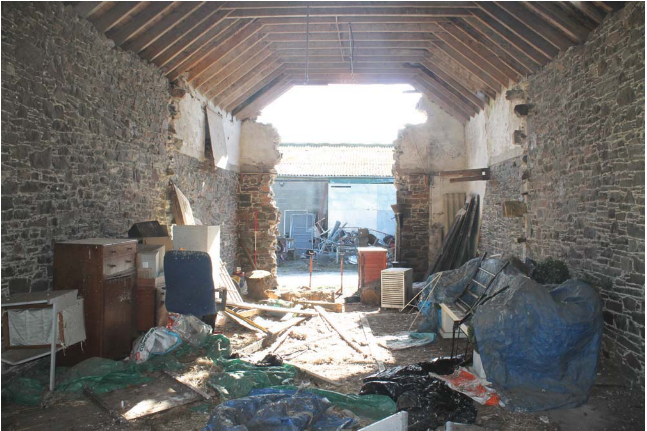
Plate 15: Barn A1/1, general view from the north
