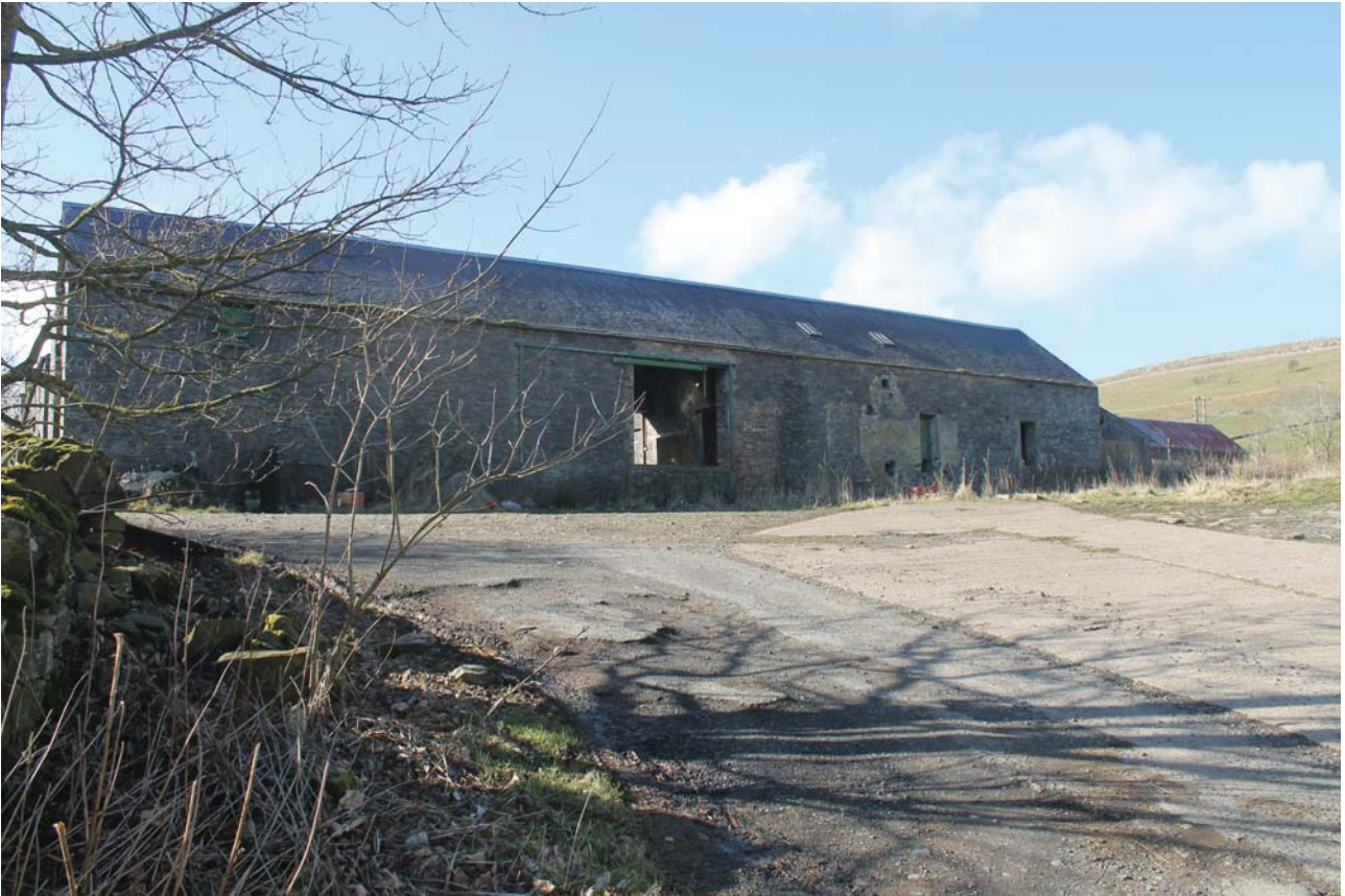
Plate 1: Barn A1, general view from the SEE
