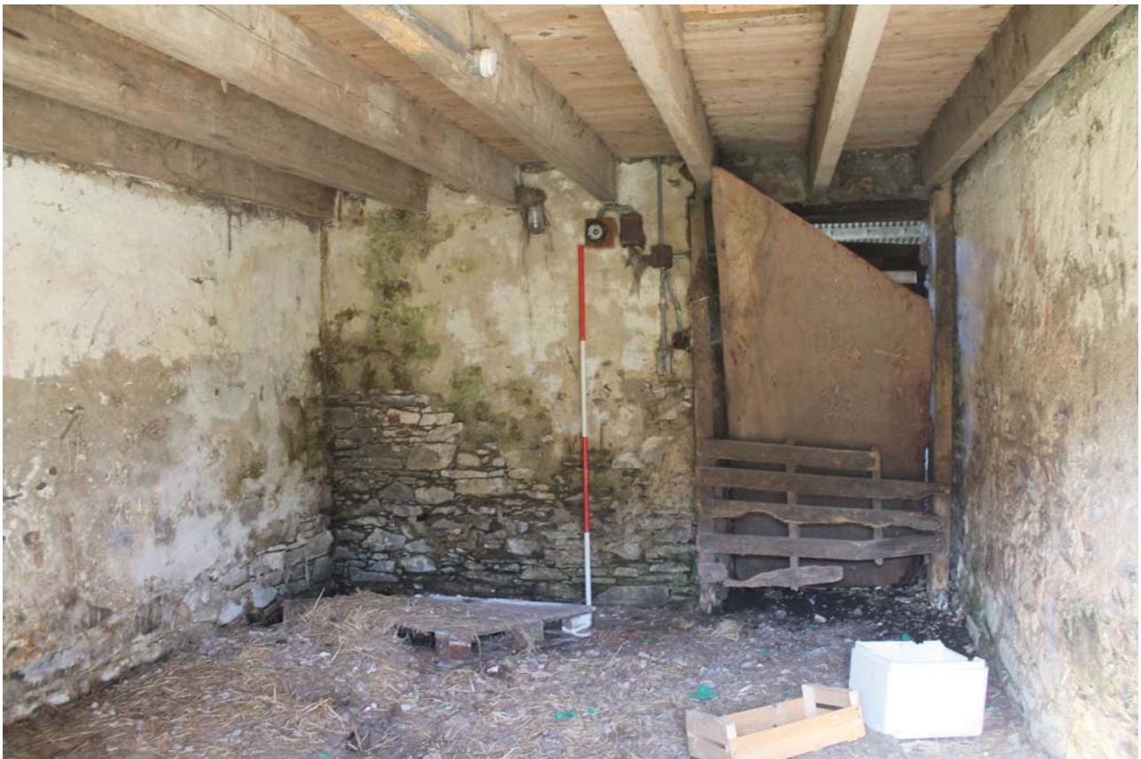
Plate 34: Barn A2/3, general view from the SSE
