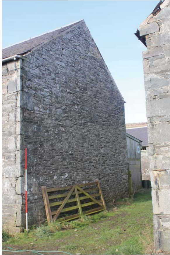
Plate 39: Barn B, east elevation, general view from the south-east
