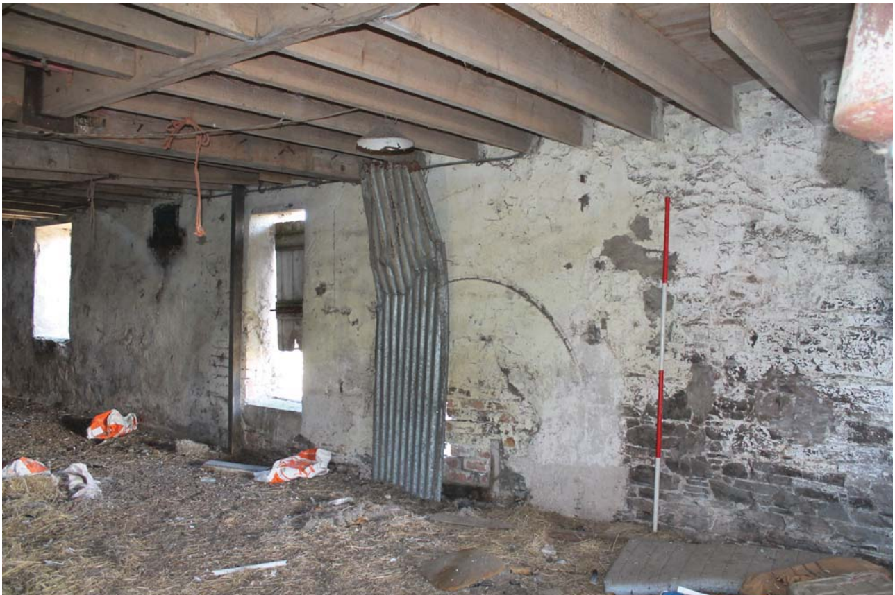
Plate 18: Barn A1/2, general view of the east wall from the south-west
