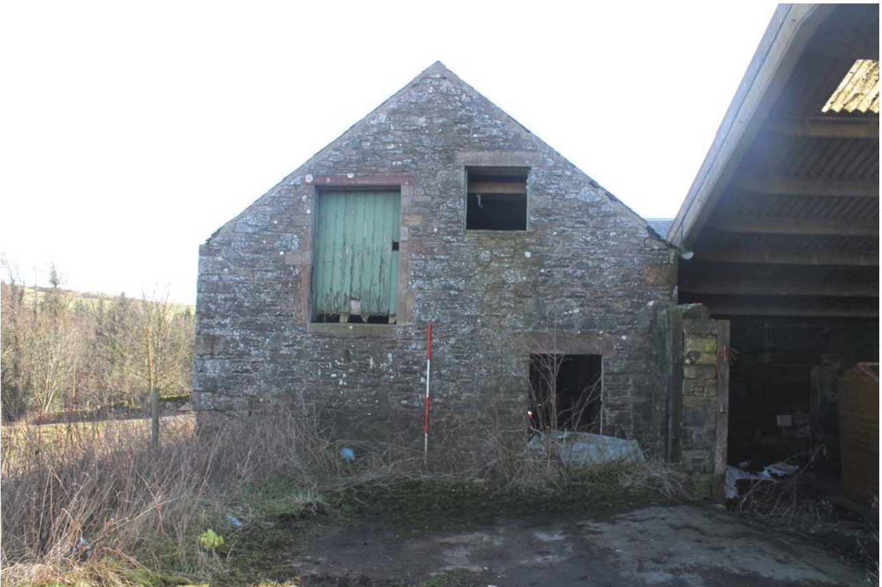
Plate 10: Barn A1, north elevation, general view from the north
