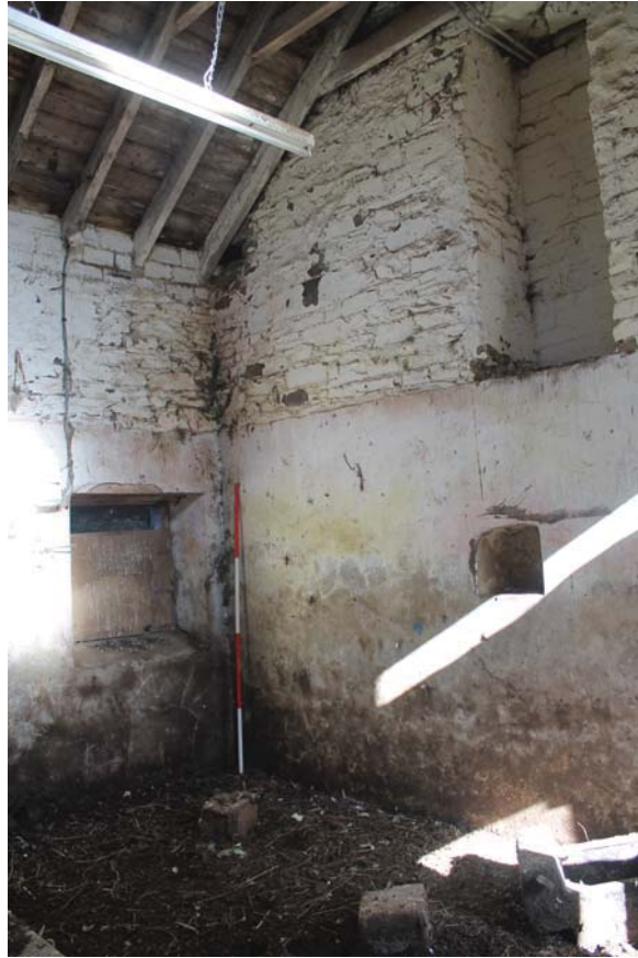
Plate 35: Barn A2/4, general view from the south-west
