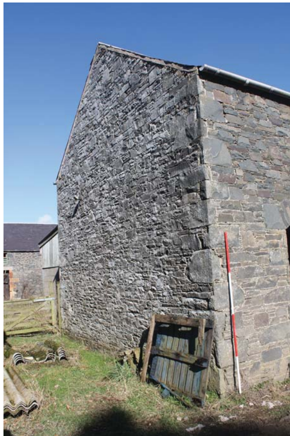
Plate 40: Barn B, west elevation, general view from the south-west
