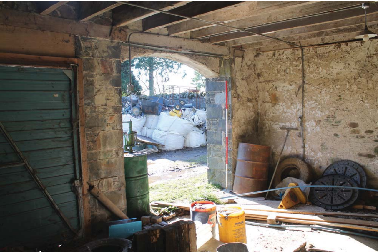
Plate 45: Barn B/2, general view from the north-east
