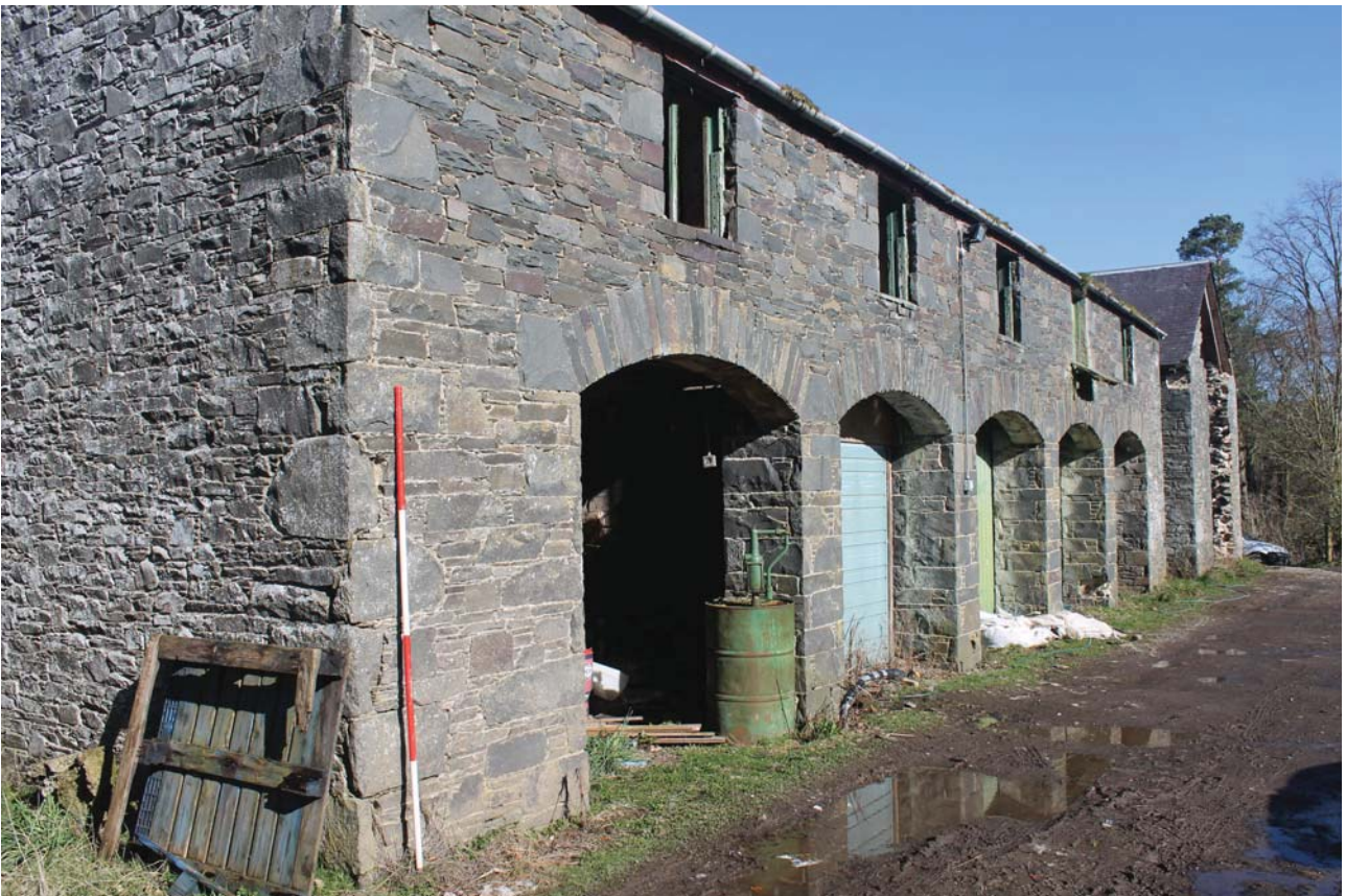
Plate 38: Barn B, south elevation, general view from the south-west
