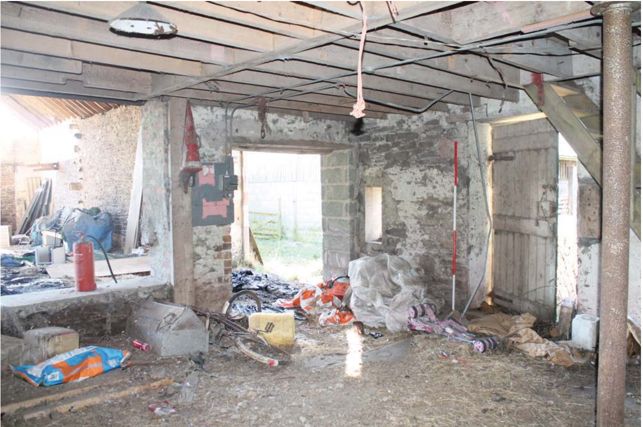
Plate 21: Barn A1/2, general view from the north-east
