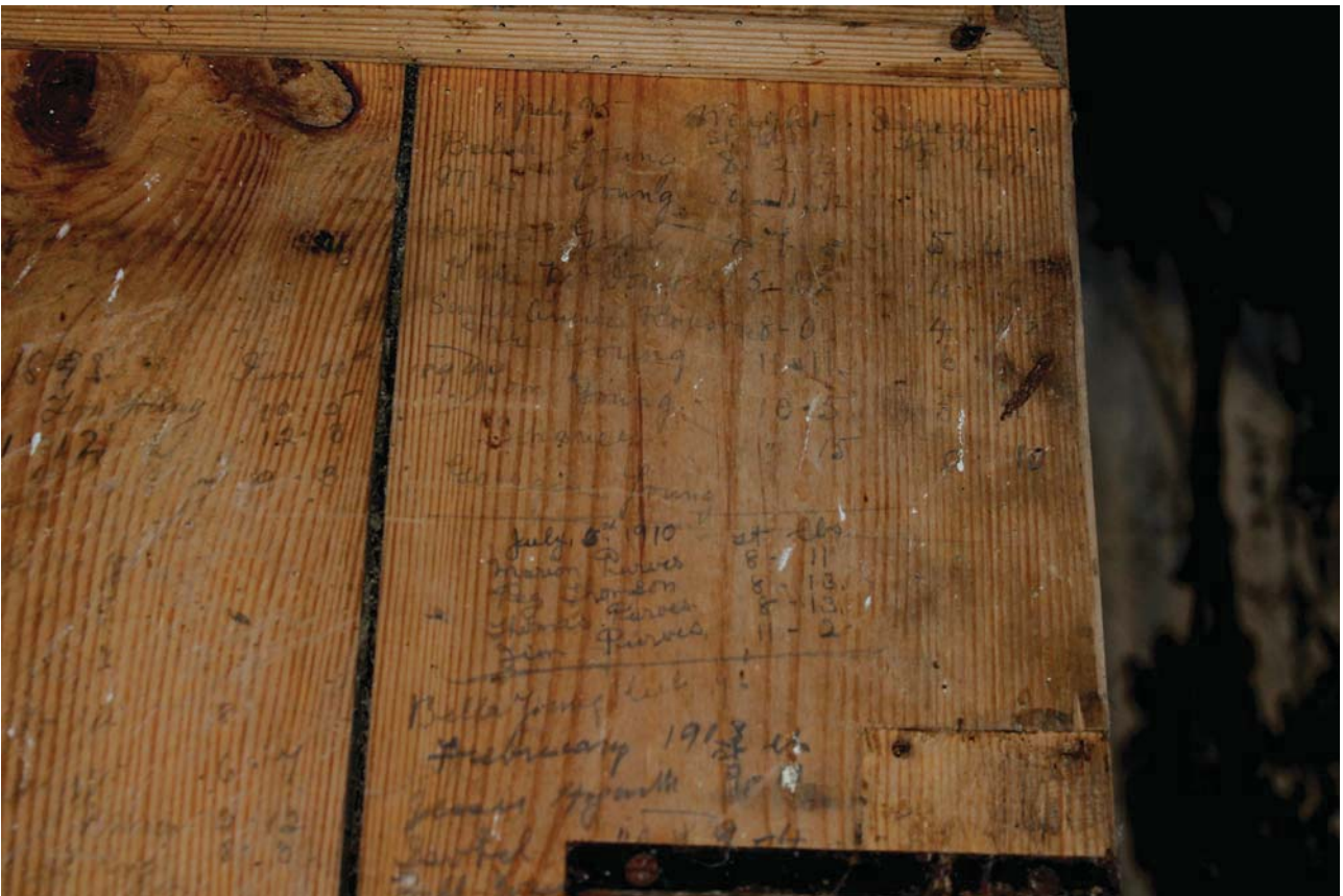
Plate 25: Barn A1/2, detail of the pencilled graffiti on the cupboard door to the west wall
