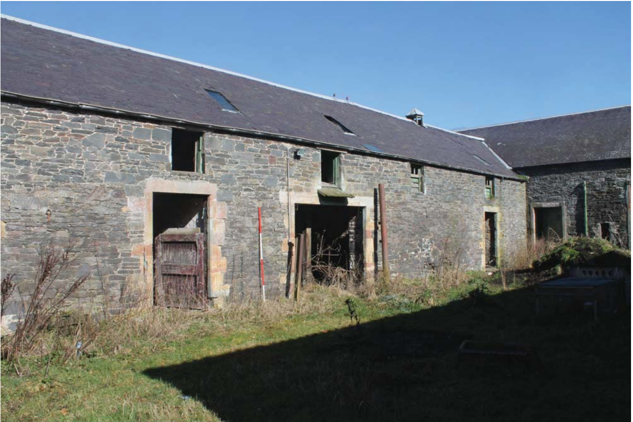
Plate 29: Barn A2, south elevation, general view from the south-west
