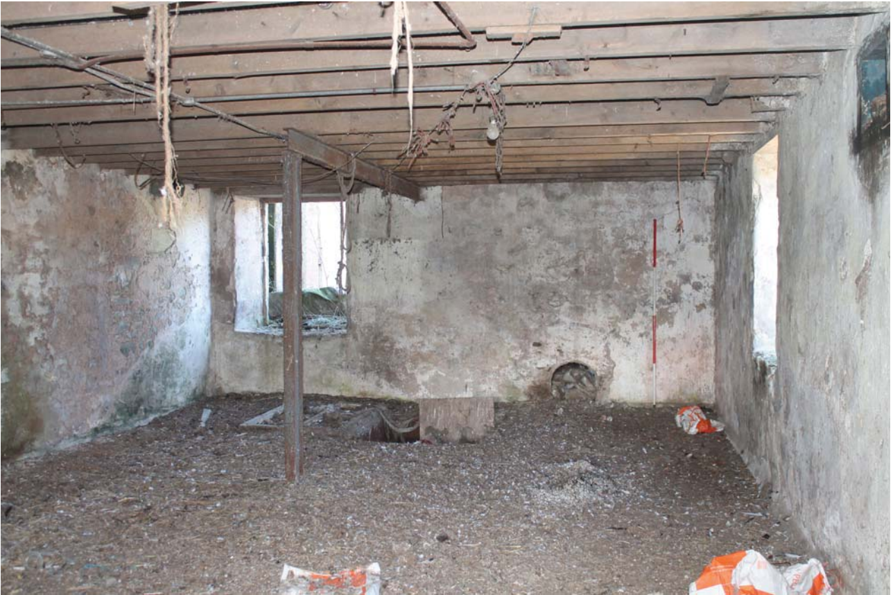
Plate 19: Barn A1/2, general view from the SSE
