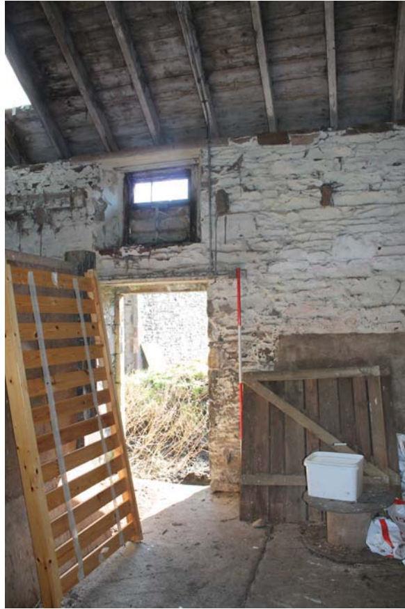
Plate 33: Barn A2/1, general view from the NNE
