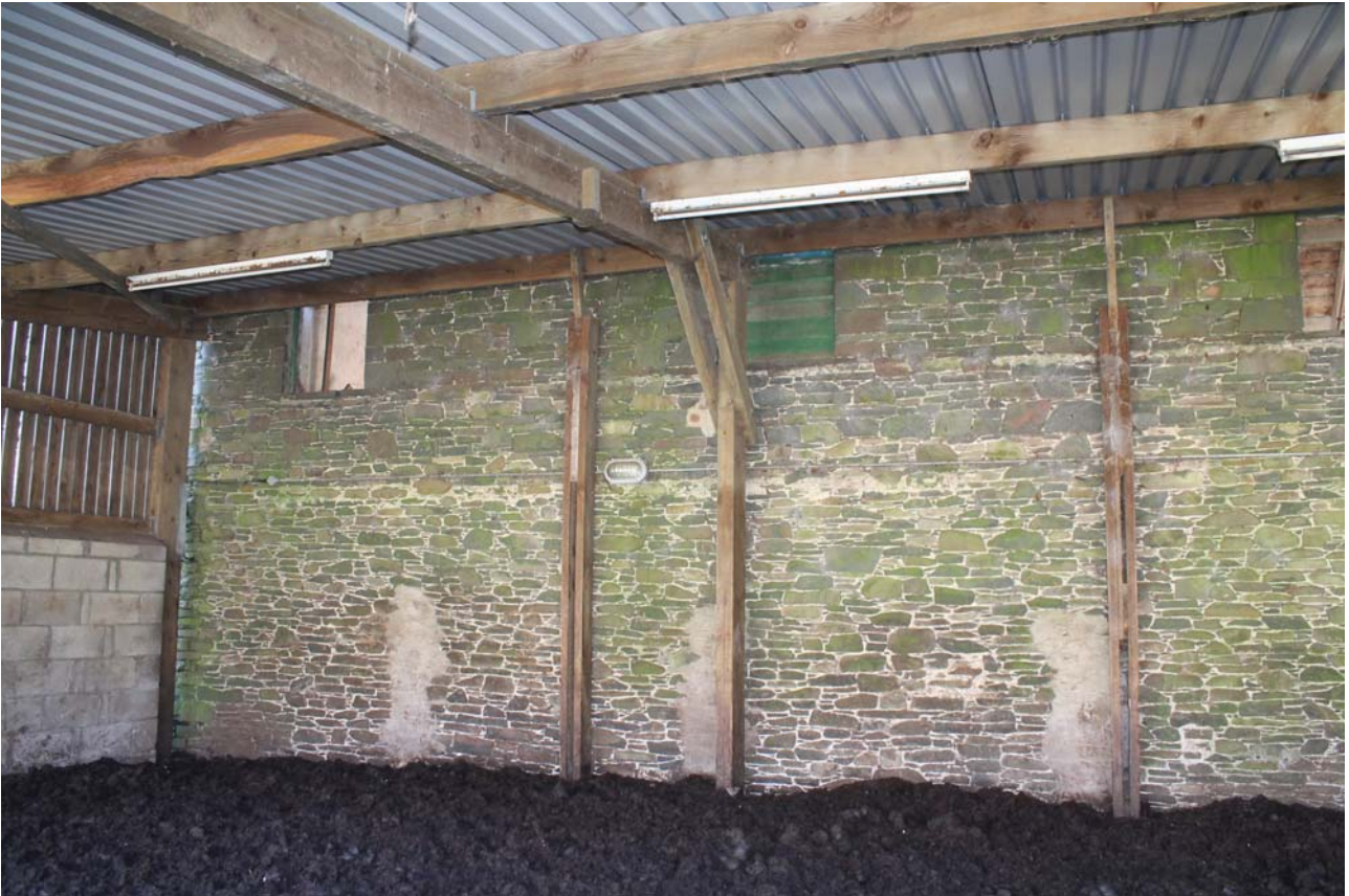
Plate 41: Barn B, north elevation, general view from the north-west
