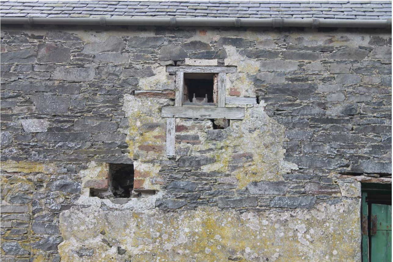
Plate 7: Barn A1, east elevation, detail of the bearing box associated with the water wheel and threshing machinery from the east
