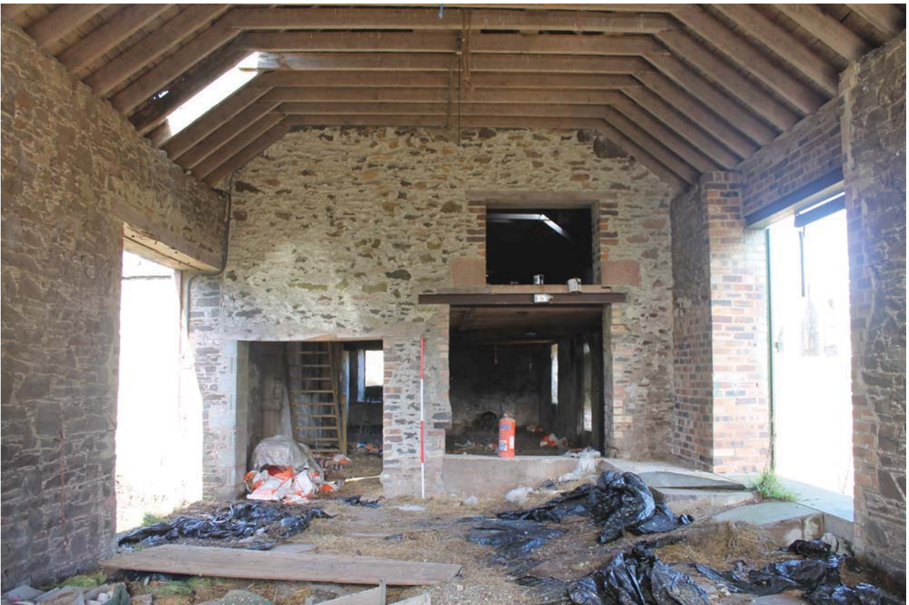
Plate 16: Barn A1/1, general view from the south
