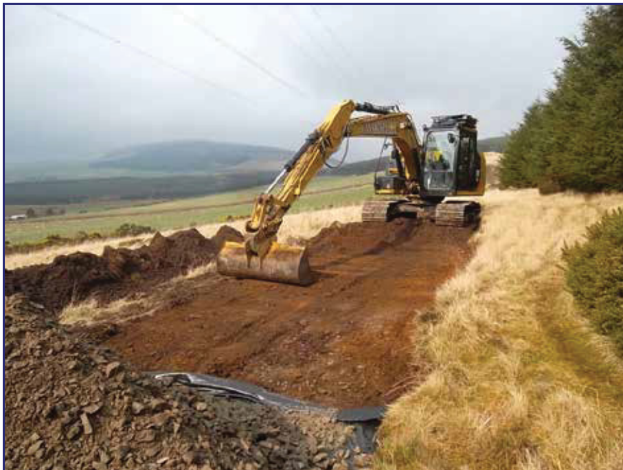
Plate 1: Access track under construction
