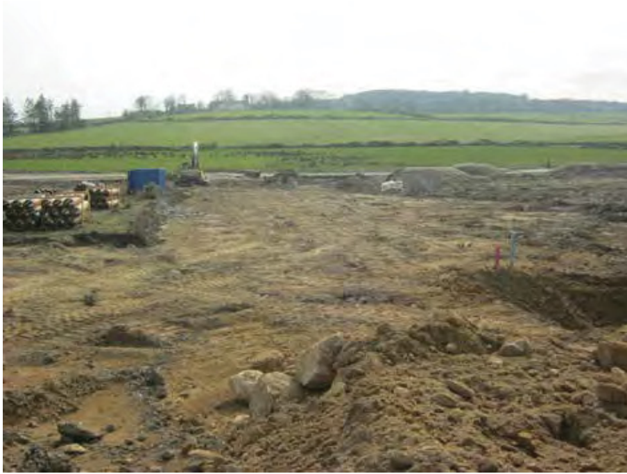
Plate 2: View of expanded Trench 7 under monitored top-soil strip
