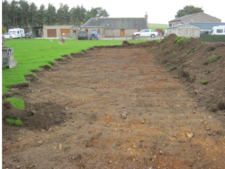
Plate 1: Area under monitored topsoil strip from east
