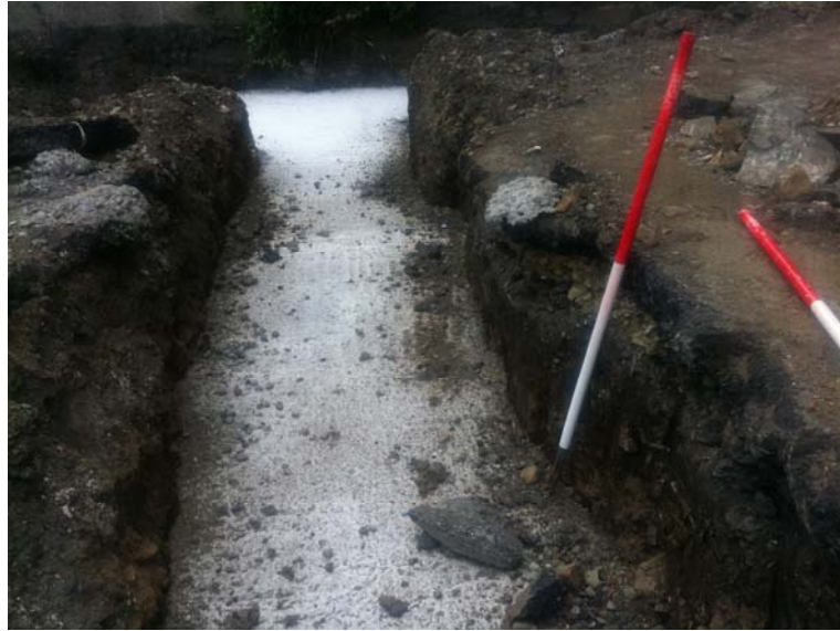
Plate 2: north east corner of area showing foundation cuts
