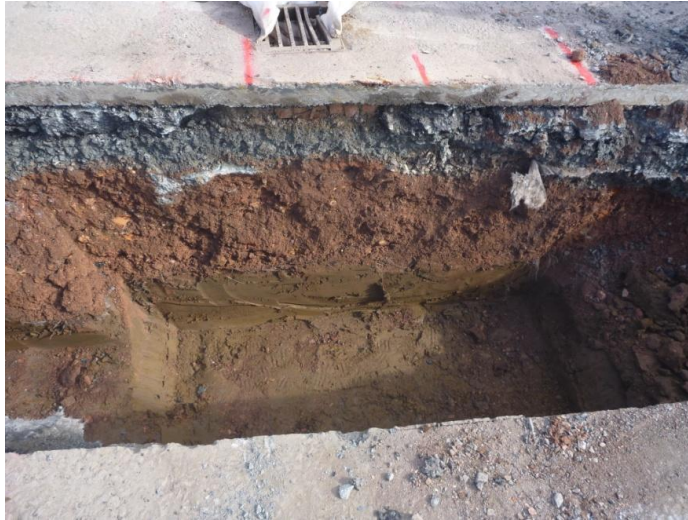
Plate 2. TR1: South-facing section showing made ground and beige clay
