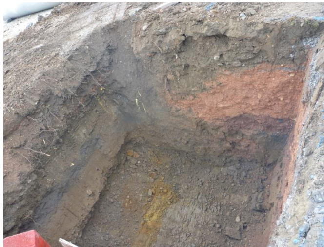
Plate 3. TR 3: East-facing section showing made ground and clay at the bottom
