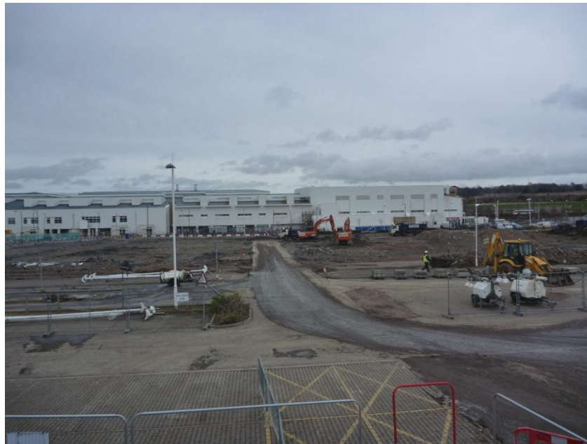
Plate 1. Site view showing area of Car Park B
