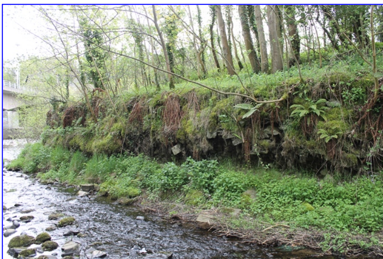
Plate 6: General view of the mill lade (northern end) from the west, showing the wall to the south side
