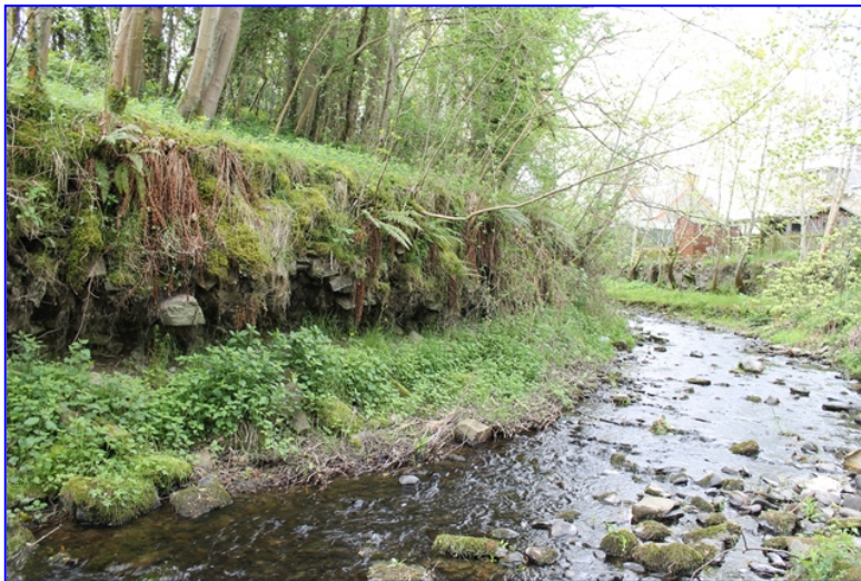
Plate 5: General view of the mill lade from the east, showing the wall to the south side (left)
