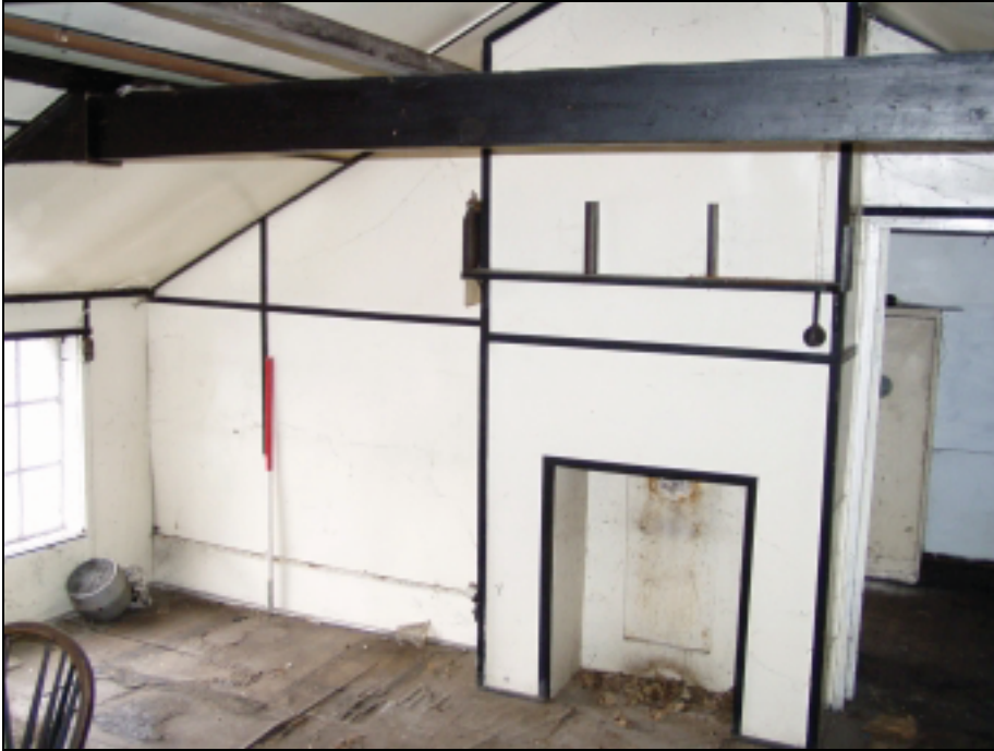
Plate 9: Fireplace First Floor, Building B
