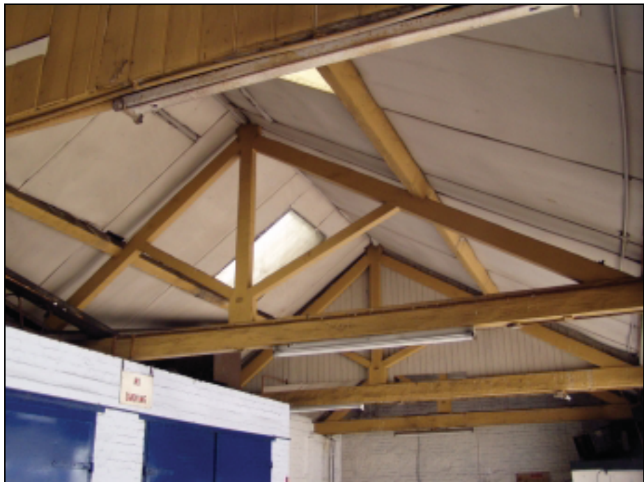
Plate 14: Roof trusses, Building D
