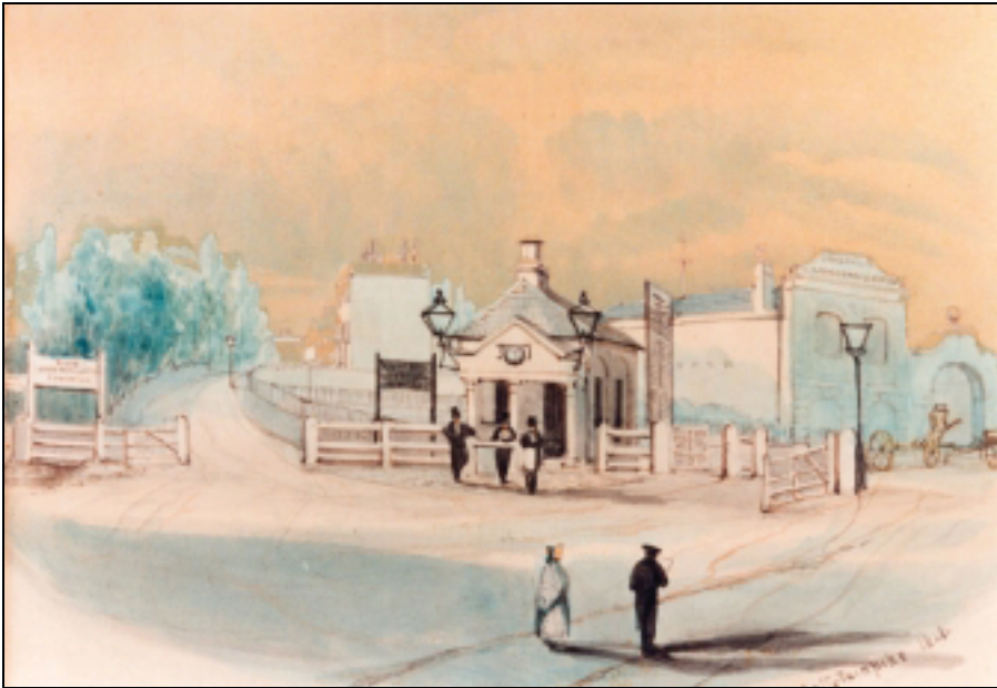
Plate 1, New Cross Toll house with 182, New Cross Road behind 1840
