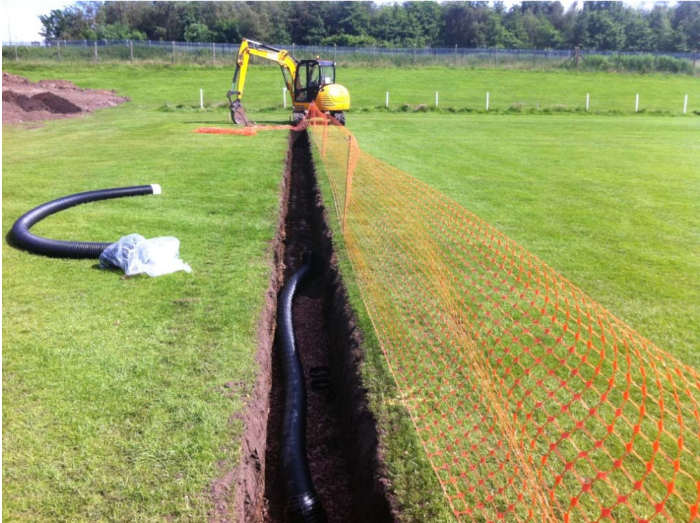
Plate 1 - General shot of main drain trench
