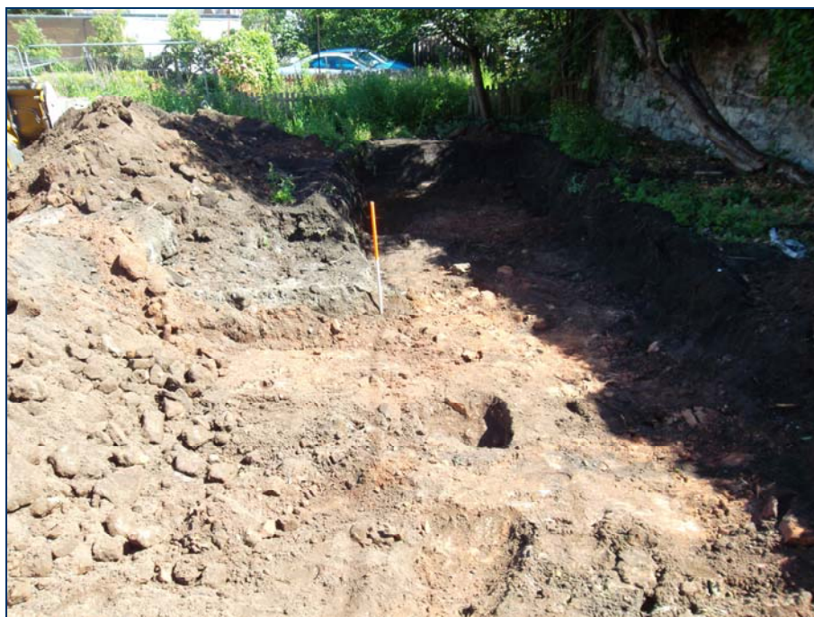
Plate 1: The area of the monitored topsoil strip, facing NE
