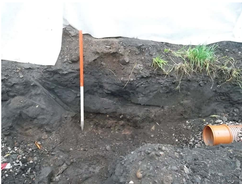
Plate 2 - Made ground in drainage trench
