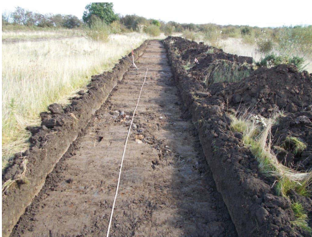
Plate 2 - Trench 30 showing rubble drain in foreground
