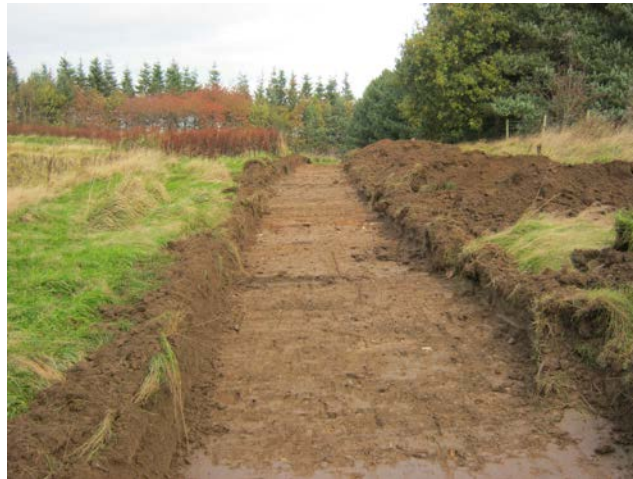
Plate 1: Trench 3 Post-excavation from south
